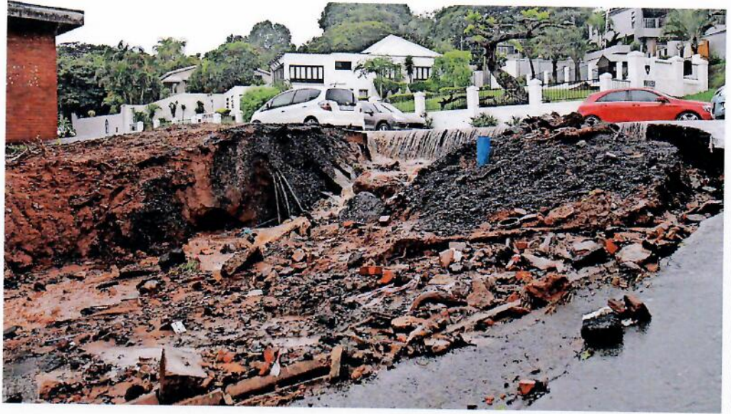
A WHOLE left hand lane is completely wiped out during a landslide caused by heavy rains in Morningside, Durban. | DOCTOR NGCOBO African News Agency (ANA)
