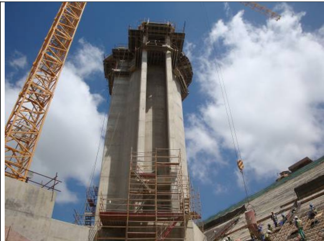
Bedford Dam under construction near Harrismith in the Free State.
