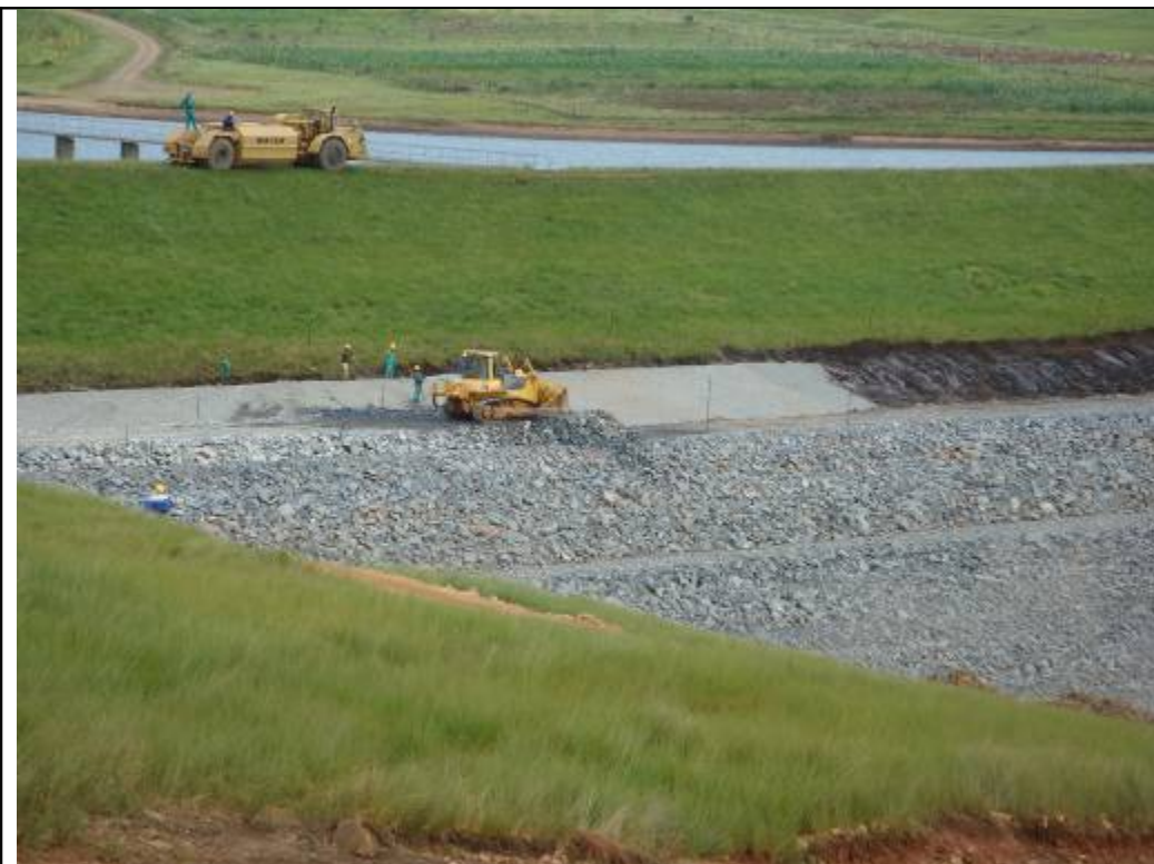
Magwa Dam in the Eastern Cape.
