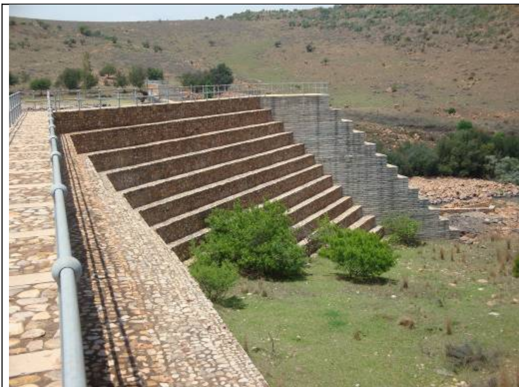
Balfour/Siyathemb a Dam near Balfour.
