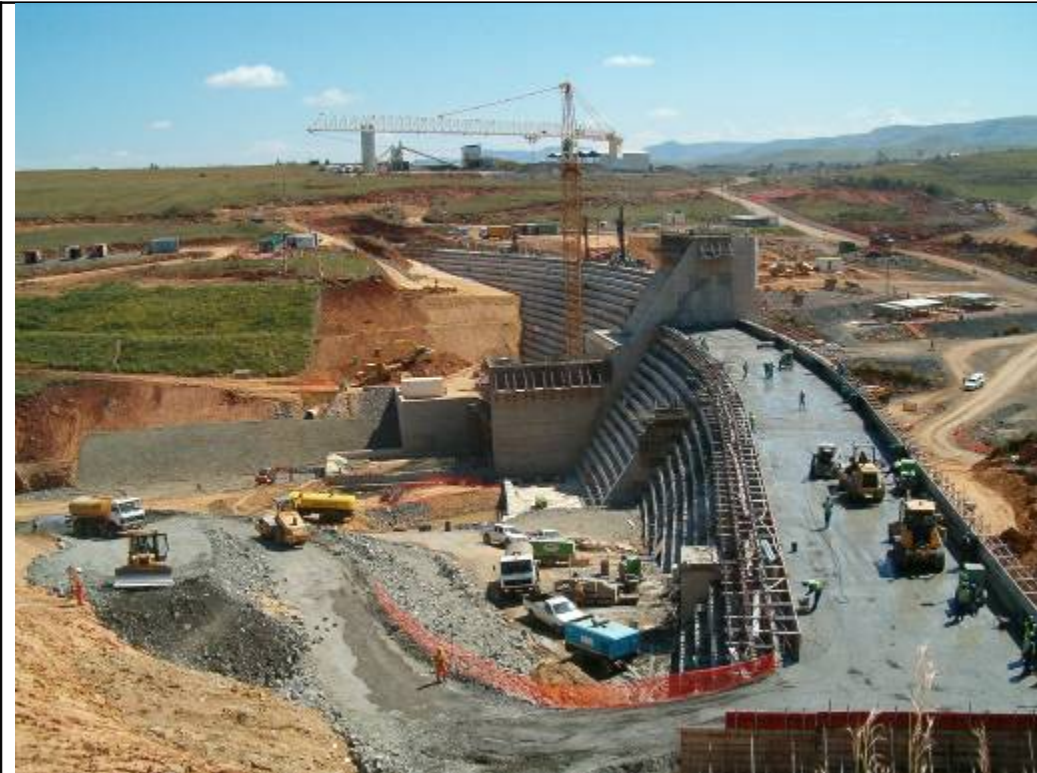
Bramhoek Dam, (gravity arch) under construction near Ladysmith in KZN.
