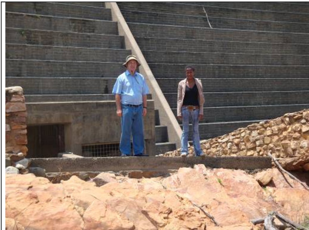
Balfour/Siyathemb a Dam near Balfour.
