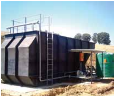
Activated sludge package plant
