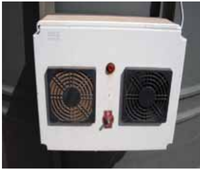
Ozonation unit at a package treatment plant
