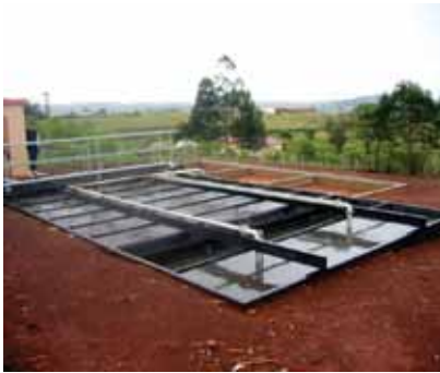
Activated sludge package plant
