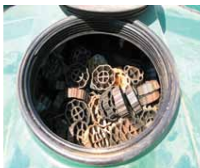
Packing material in a submerged bio-contactor – Note that the shape and size of the packing may vary with different units
