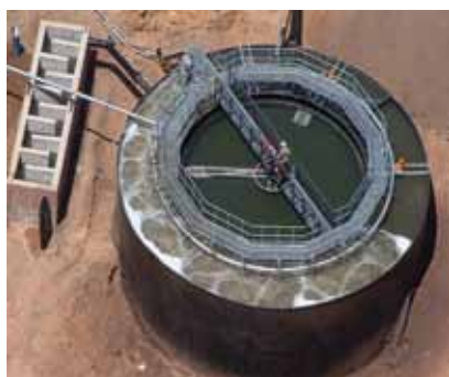
Extended aeration installation
