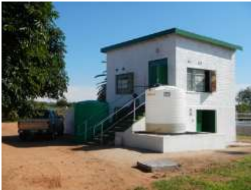
Seshego WTW is a neat & well-maintained facility
