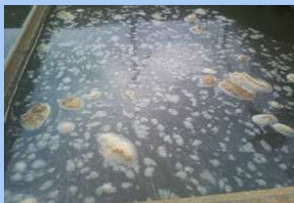
Scum accumulation in flocculation channels is evident
