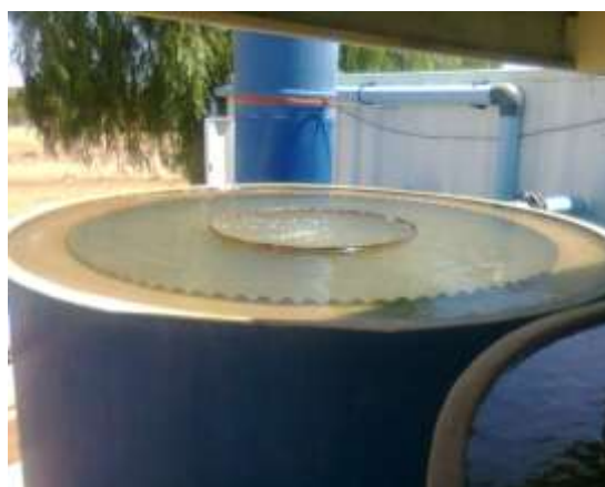
Overflowing clarifier at Boegoeberg WTW
