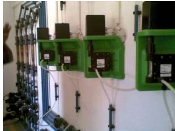
Good condition of chlorinators
