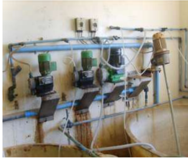
Dosing pumps at the Kakamas WTW
