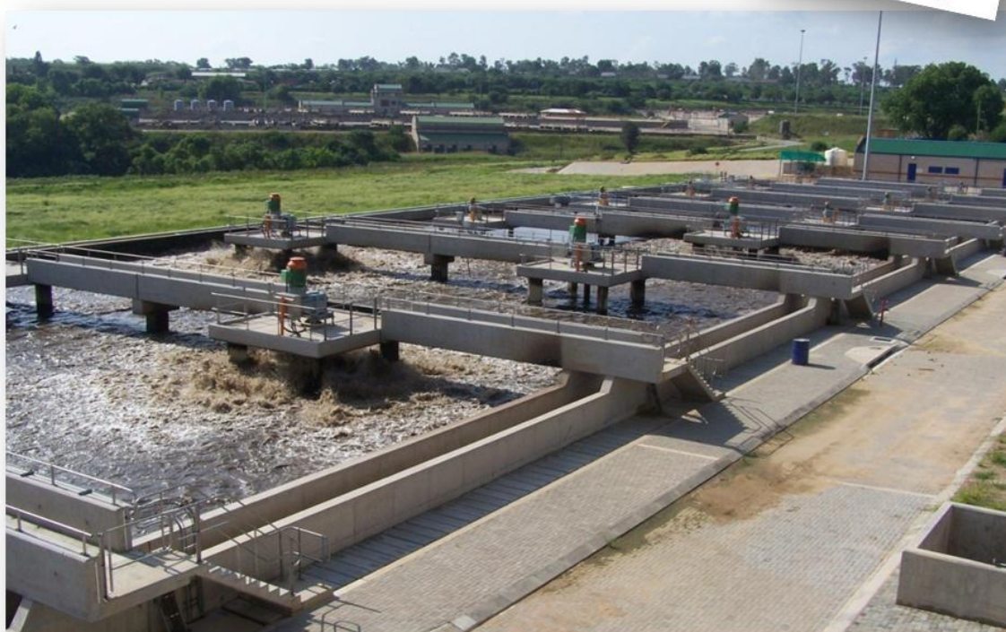
Johannesburg Northern Works – achieving excellent biological phosphate removal and revert to chemical dosing as a secondary measure.
