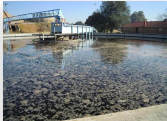
Left: unmaintained sludge drying beds; Right: scum formation on the secondary clarifiers under overload conditions
