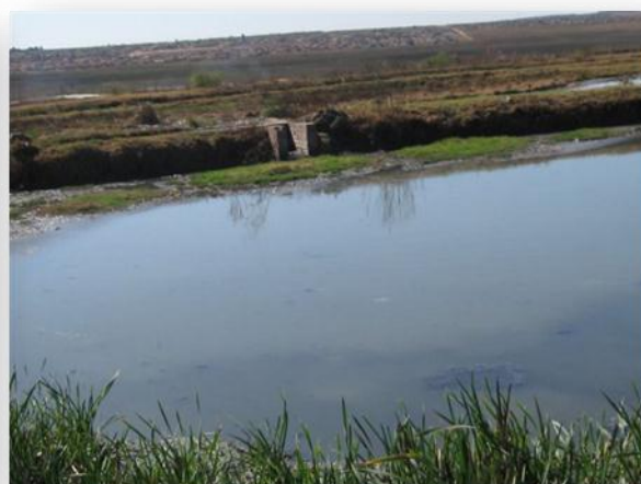
Sludge accumulation in the pond system, highly overloaded
