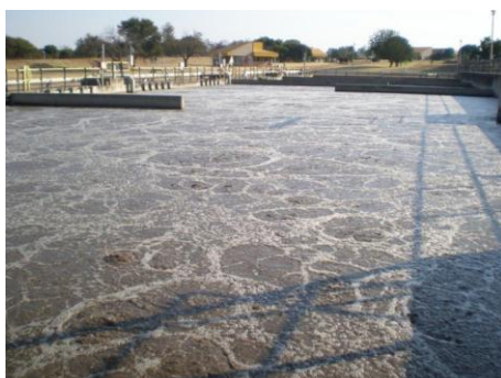
Left: sludge carry over at the sludge settling tanks; Right: ponds filled to capacity at the Rooiwal plant
