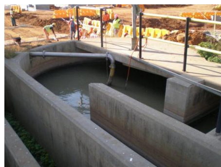
Left: sludge carry over at the sludge settling tanks; Right: ponds filled to capacity at the Rooiwal plant
