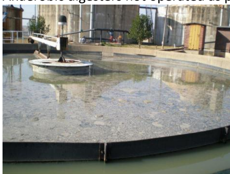
Left: sludge carry over at the sludge settling tanks; Right: ponds filled to capacity at the Rooiwal plant
