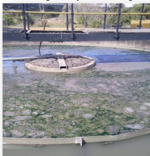
PST has not been desludged for an extended period, due to breakdown of sludge pumps. Sludge build-up is compromising the down-stream treatment units
