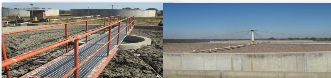
Unmaintained state of primary settling tanks (left) and dysfunctional (newly constructed) biofilter (right) - result in substandard effluent quality being discharged to the receiving environment
