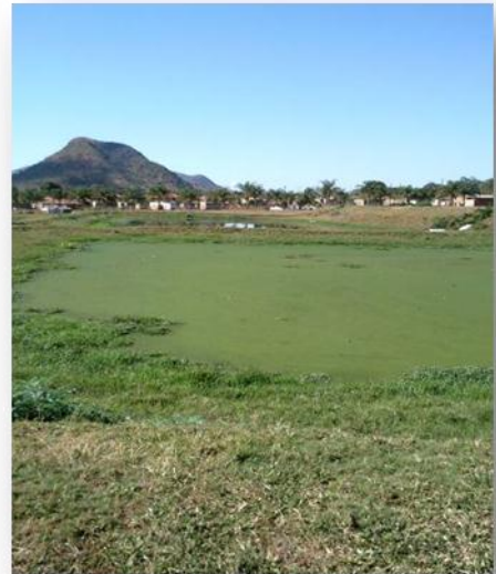
4 of 7 ponds operational – overloaded and producing poor effluent quality at point of discharge – pipes between ponds broken
