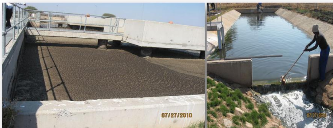
Inadequate process control, with severe scum formation and short circuiting in the anaerobic basin of the activated sludge reactor
