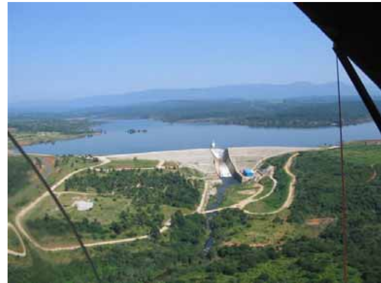
Inyaka Dam after Construction
