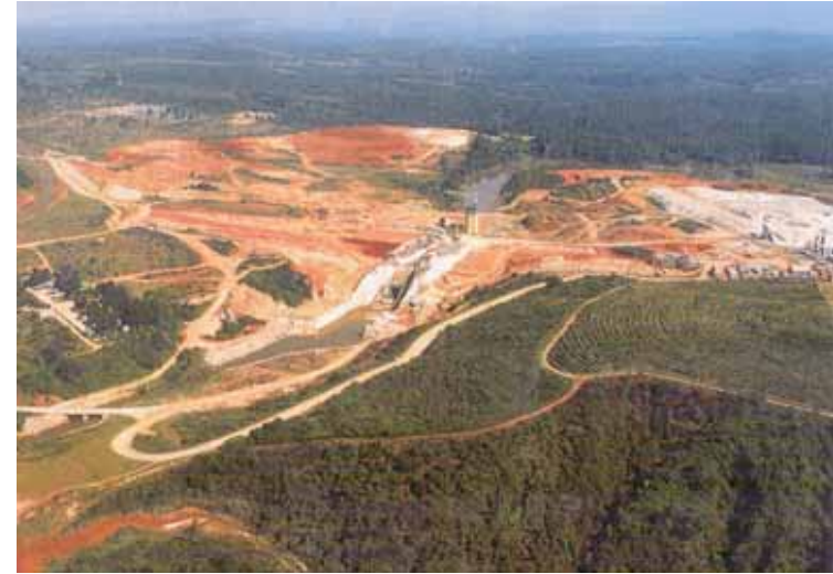
Inyaka Dam during Construction
