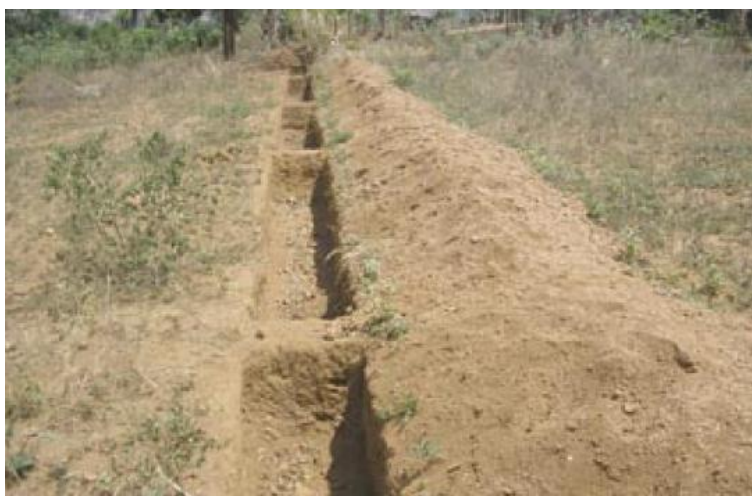
Figure 53 Lock-and-spill ditch for catchment protection, Rwanda (Mati, 2008)
