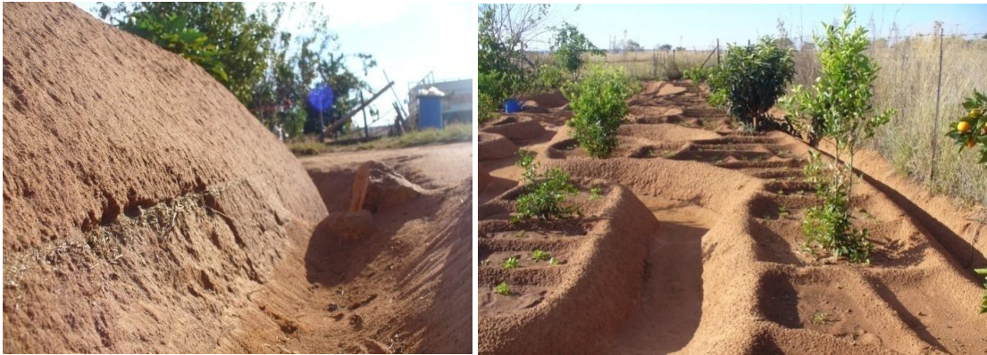
Figure 39 Water marks showing the level of ponding in the bottom ditch before overflowing downhill (towards the right on the photo) during a rainstorm. Infiltration into the ridge on the left produced a bumper crop of sweet potatoes, which had just been planted into the ridge at the time of this photo (WRC, 2010)
