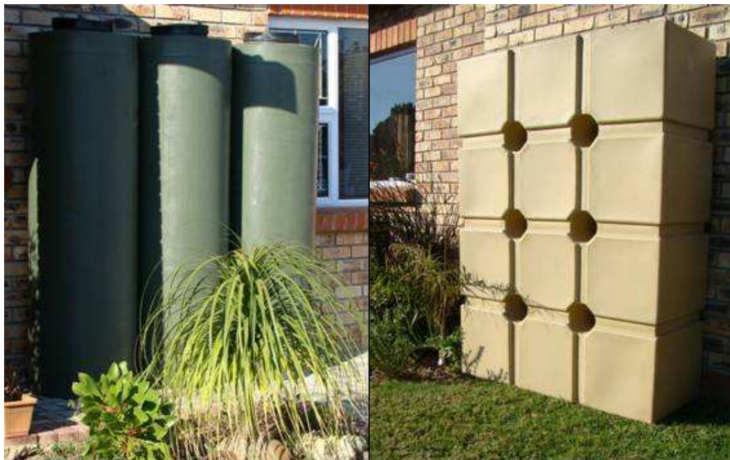
Figure 1 Rainwater storage tanks
