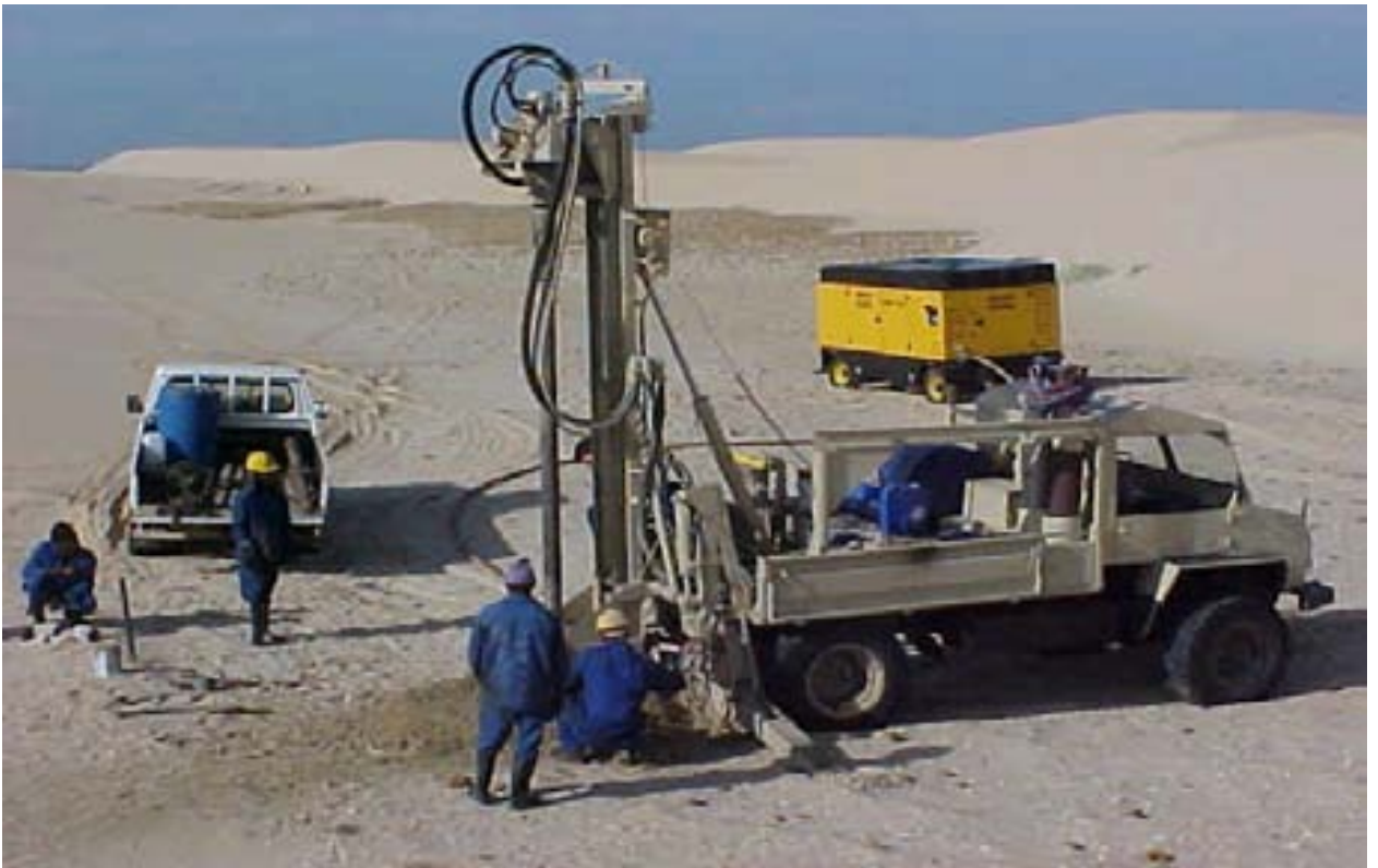
Plate 15: Dune Aquifer Exploration Drilling
