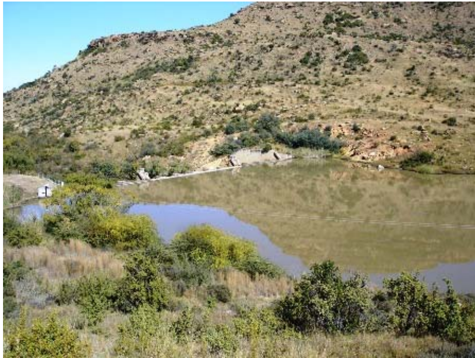
Figure 3: Meulspruit Dam. The Meulspruit is a tributary to the Caledon River, downstream of the town Ficksburg.
