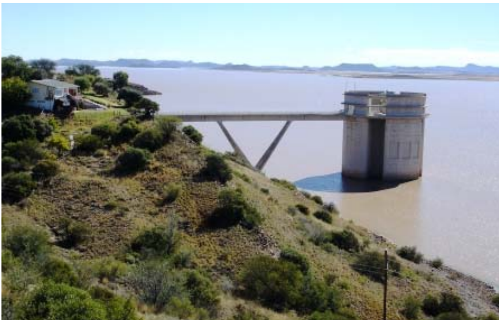
Figure 8: Oviston inlet tower situated on Gariep Dam.
