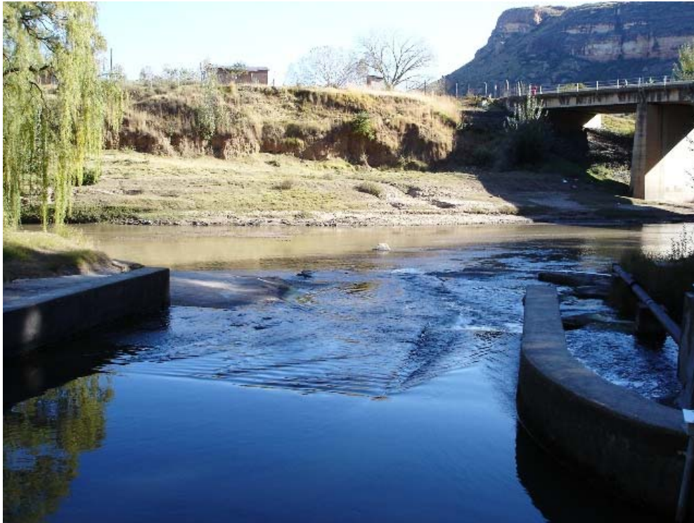
Figure 2: Gauging weir on the Caledon River, at the confluence with the Little Caledon River.
