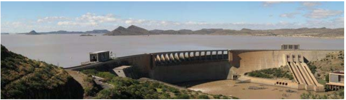
Figure 7: The impressive Gariep Dam Wall
