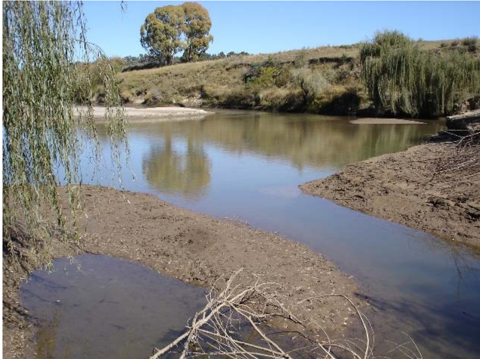
Figure 4: Caledon River upstream of Ficksburg (bordering with Lesotho) showing partially eroded banks and the consequences of high sedimentation rates.
