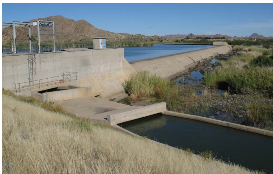
Figure 23: Northern bank canal at Neusberg weir close to Kakamas.
