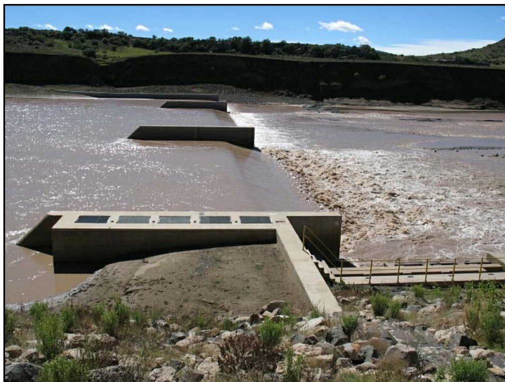
Figure A1: A) Satellite image (Google Earth) and B) on site picture of the new gauging weir at Oranjedraai (OS1). River width at weir was approximately 160 m.
