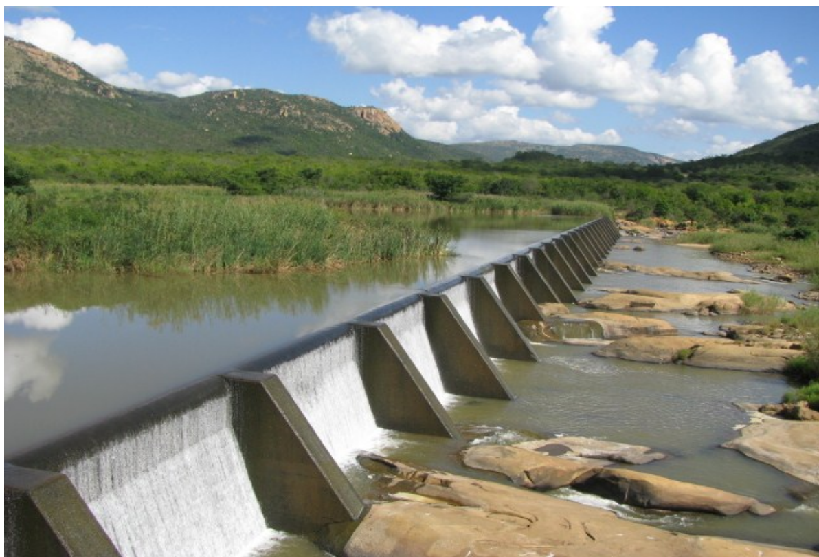
Photo 5.1: Photo of the Grootdraai weir illustrating build-up of sediment
