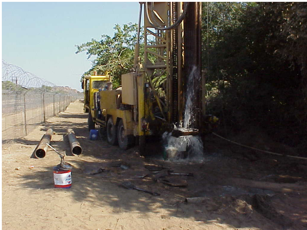
Figure 7: Drilling boreholes
