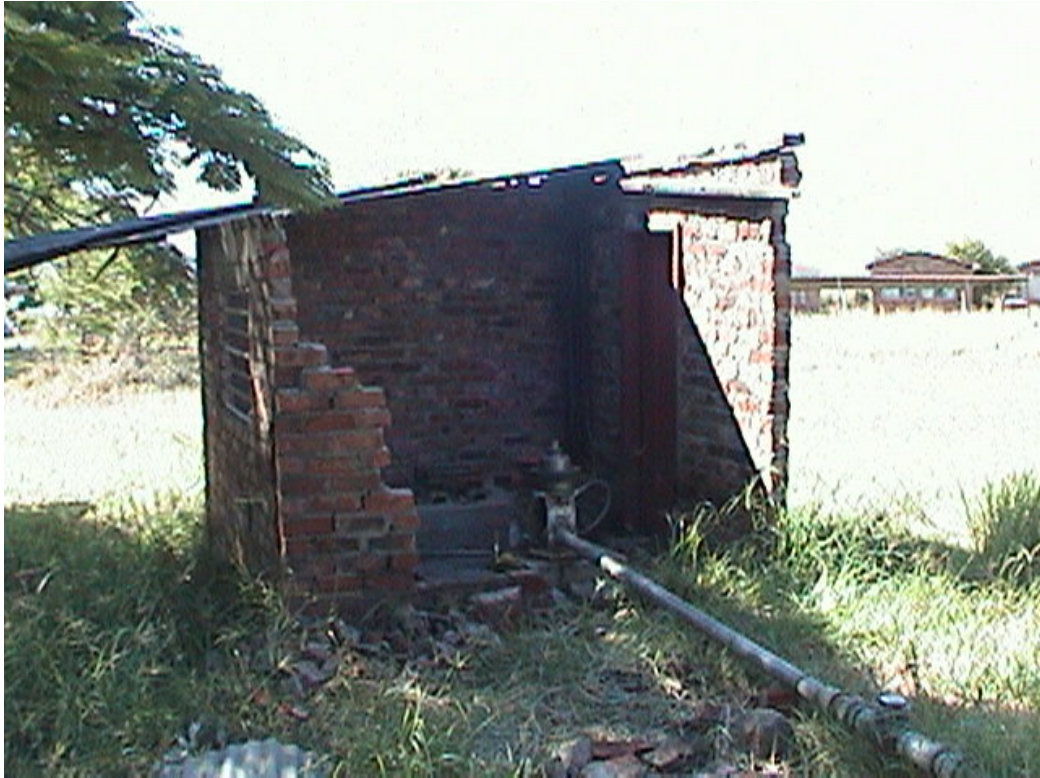
Figure 4: Destruction of borehole infrastructure affects reliability of supply
