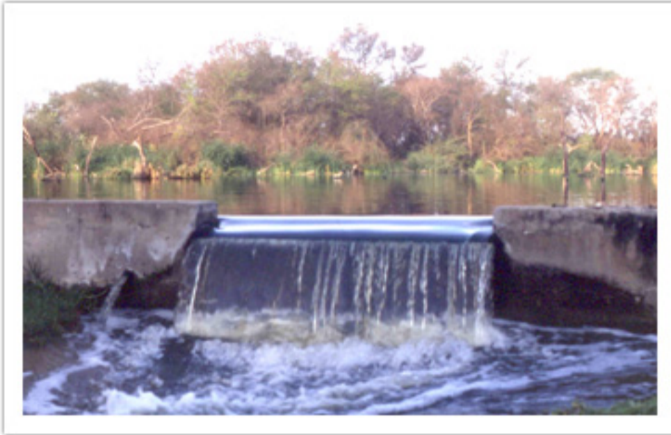
Photo 2: Polokwane's artificial recharge water source - discharge of treated waste water from the final maturation pond
