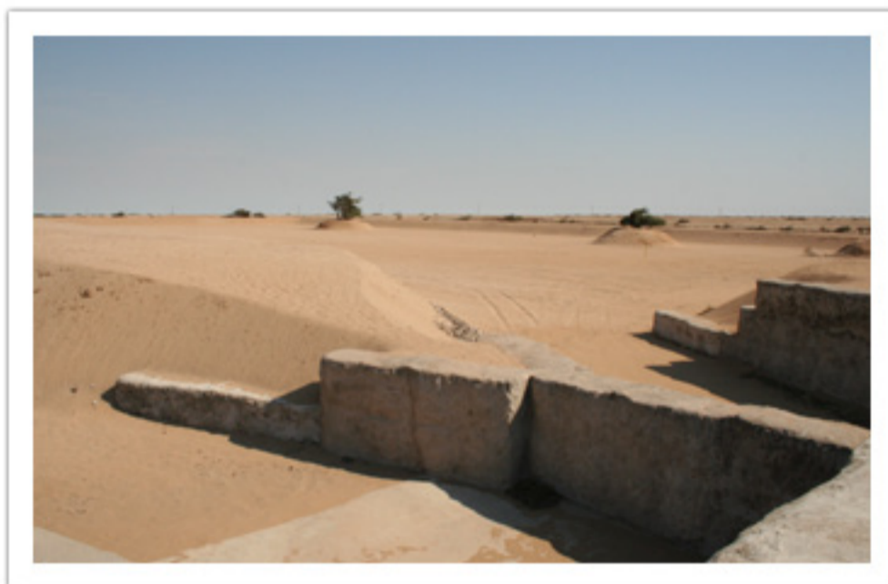
Photo 6: One of Omdel's infiltration basins
