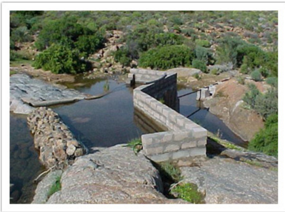
Photo 4: Kharkams' in-stream sand filter. Water is led from here to the injection boreholes.
