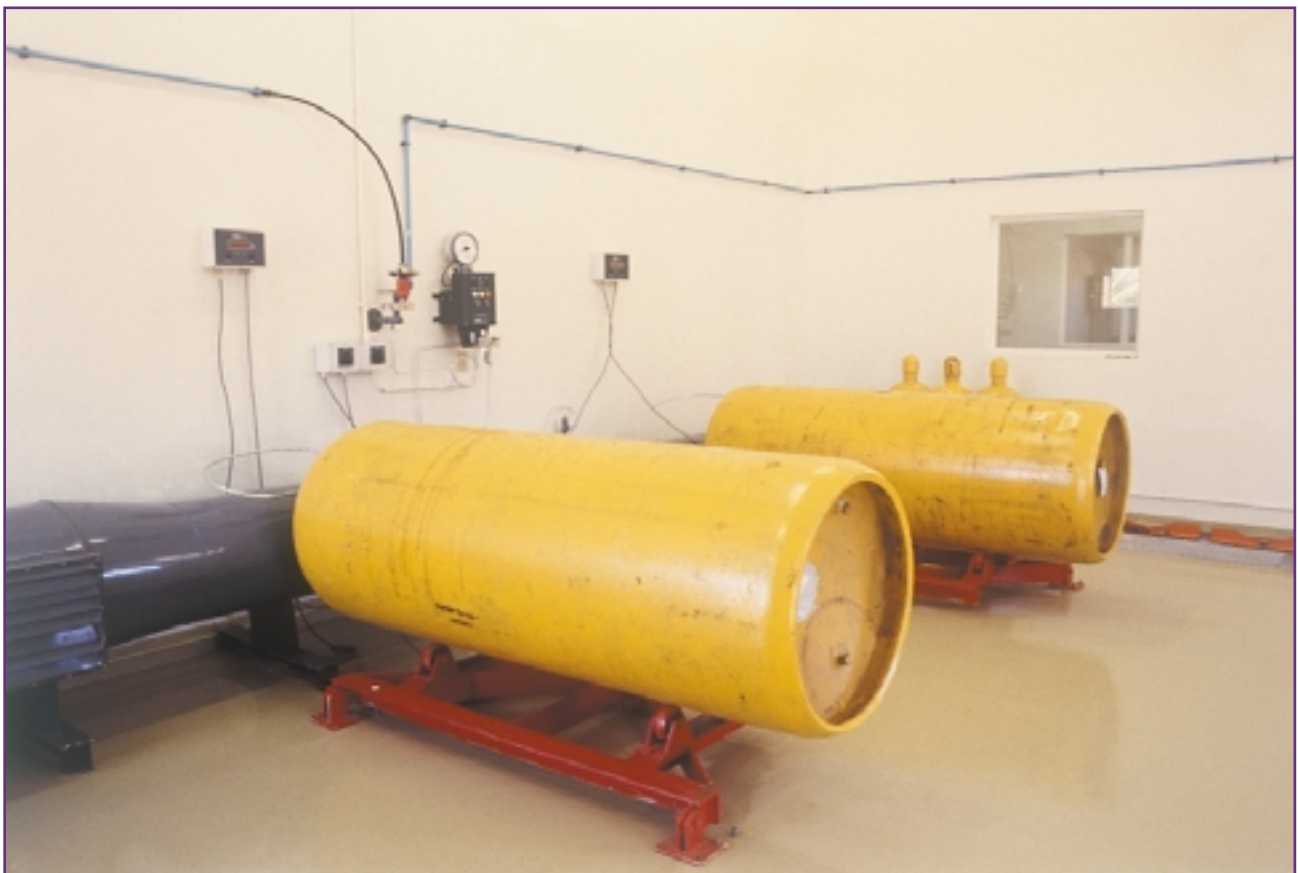
Figure 15: Chlorine cylinders providing chlorine gas for disinfection of water
