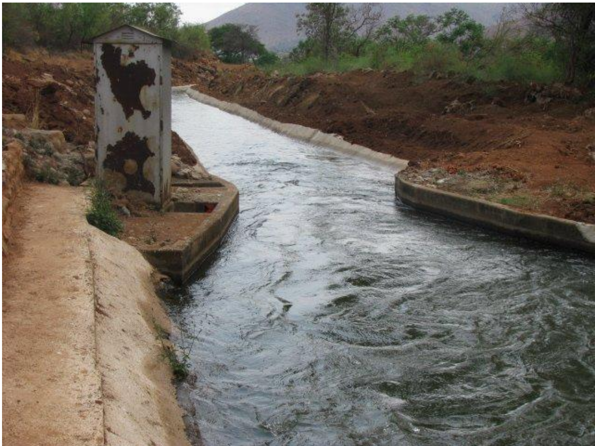
Figure 3-7: Measuring structure at inlet to the scheme
