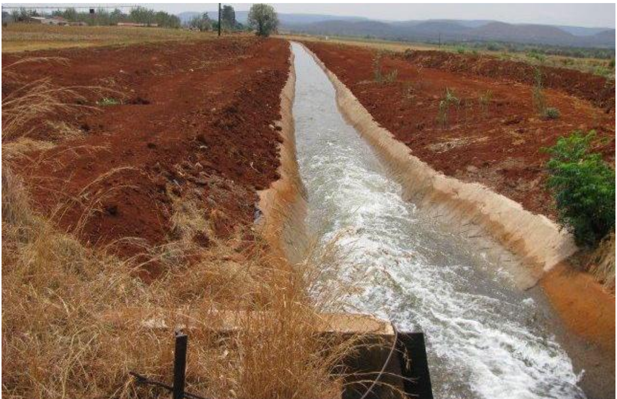
Figure 3-5: View of lined canal
