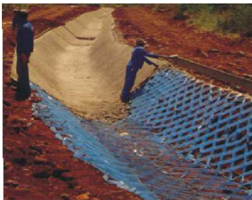
Figure 3-3: Use of Hyson cells during construction
