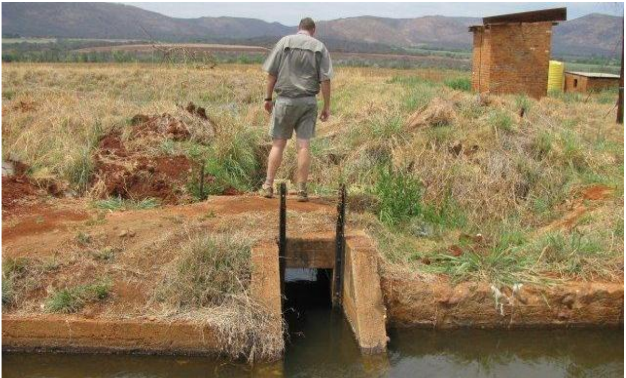
Figure 3-4: Sluice at property
