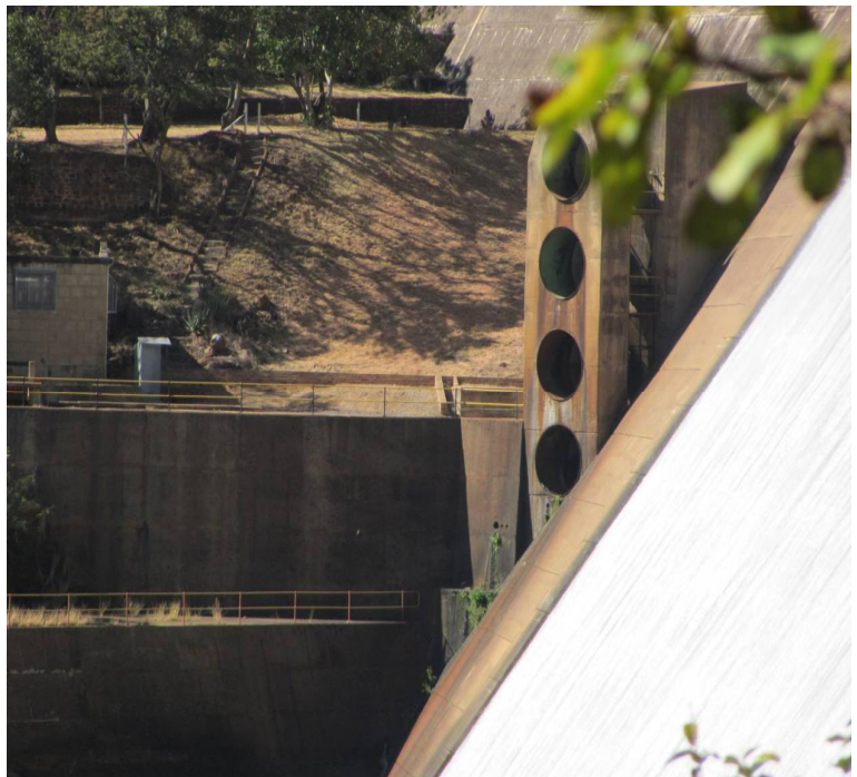
Figure 3-2: Outlet works at Loskop Dam
