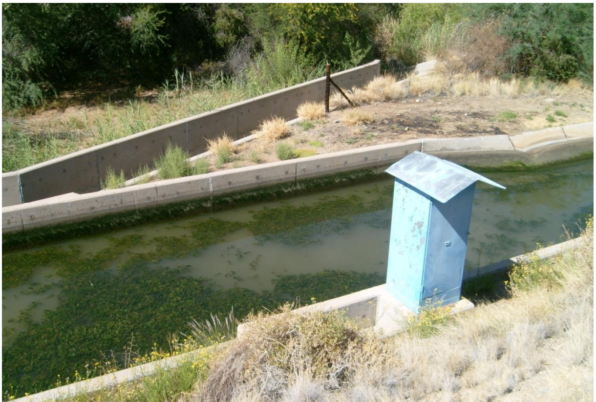
Figure 3-7: Measuring point at reject structure
