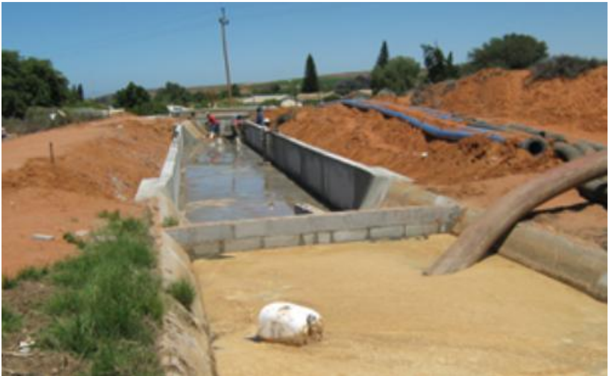
Figure 7-5: Lutzville canal break - reparation in progress
