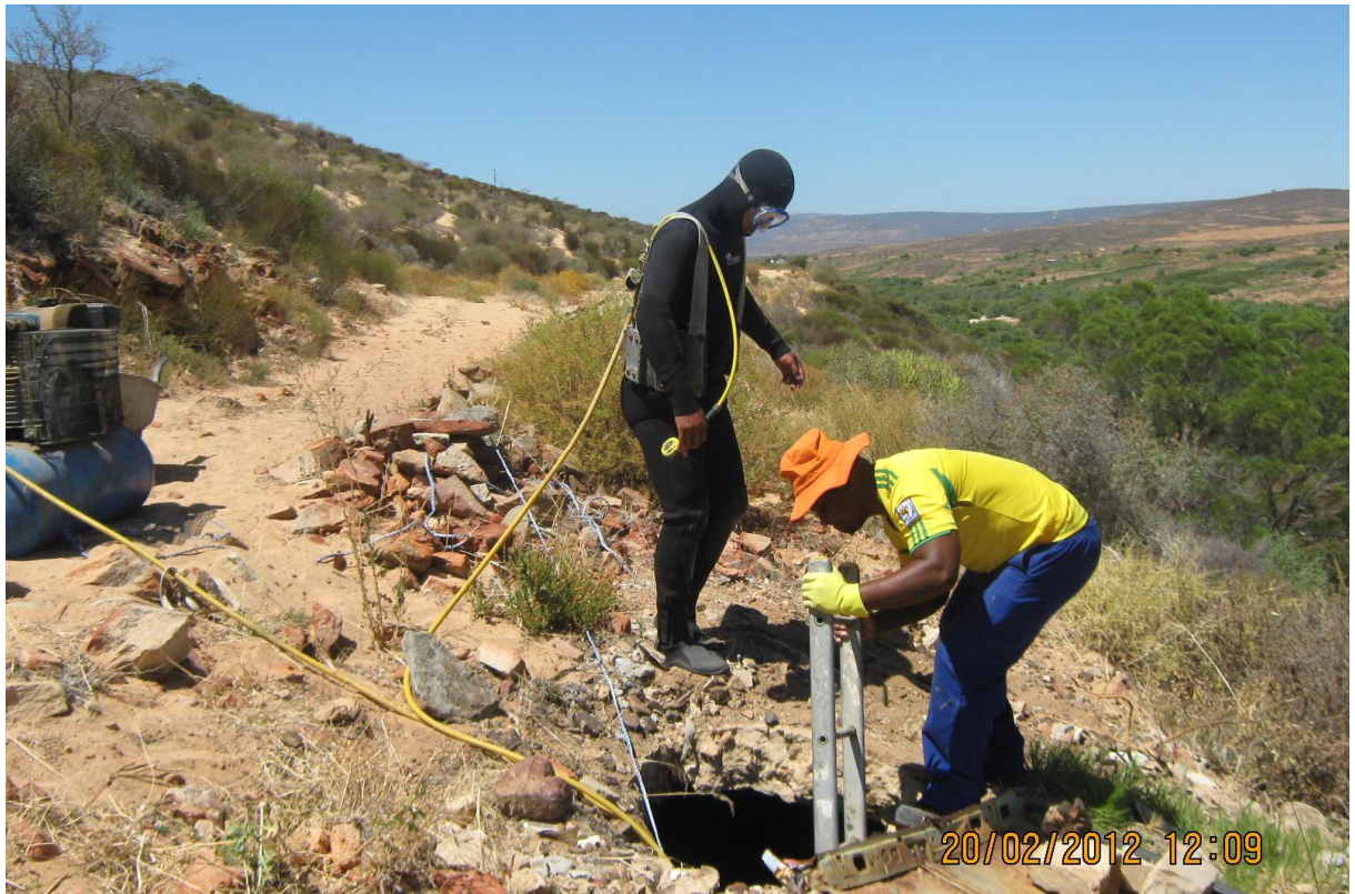
Figure 7-1: Diver preparing to undertake maintenance in closed canal
