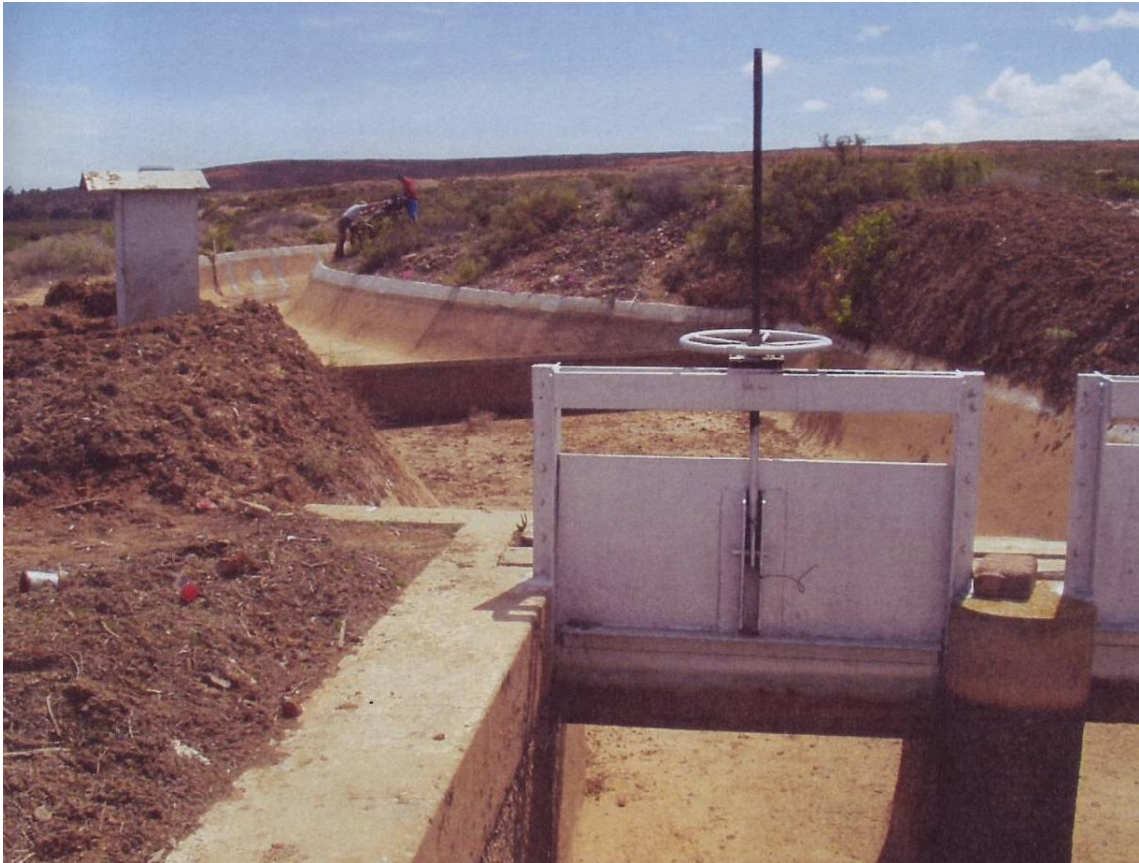
Photo 3-2: Sharp-crested measurement structure for Koekenaap section
