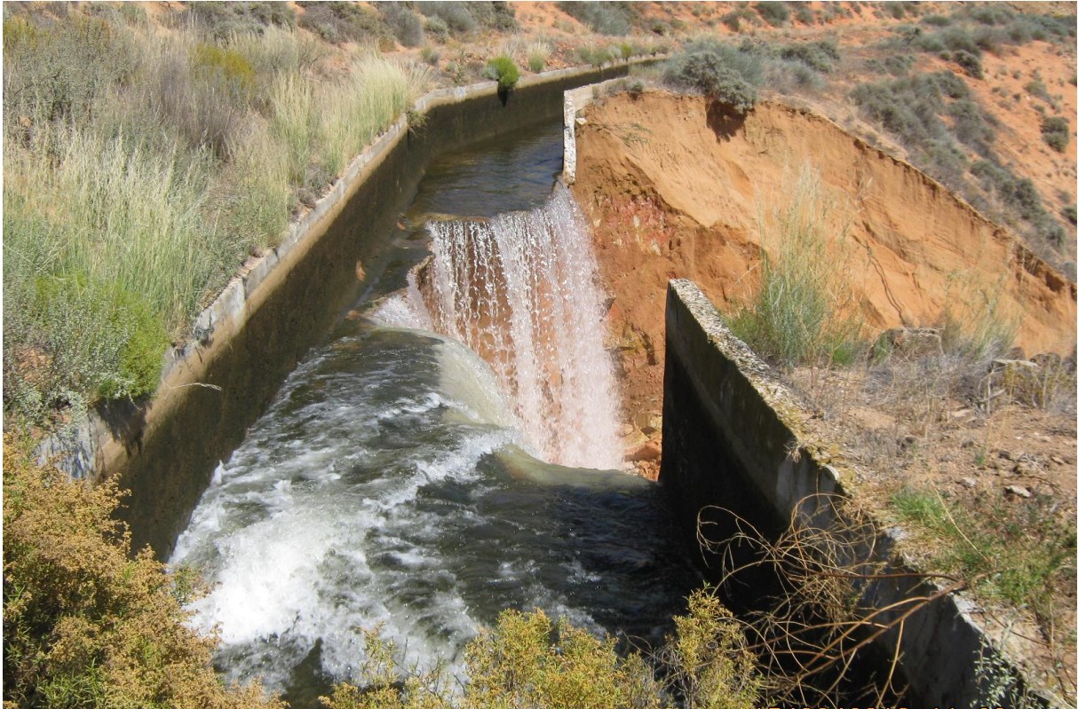
Figure 6-3: Canal break
