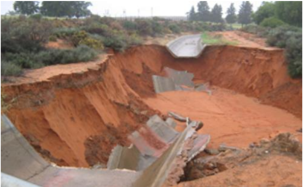
Figure 7-4: Lutzville canal break
