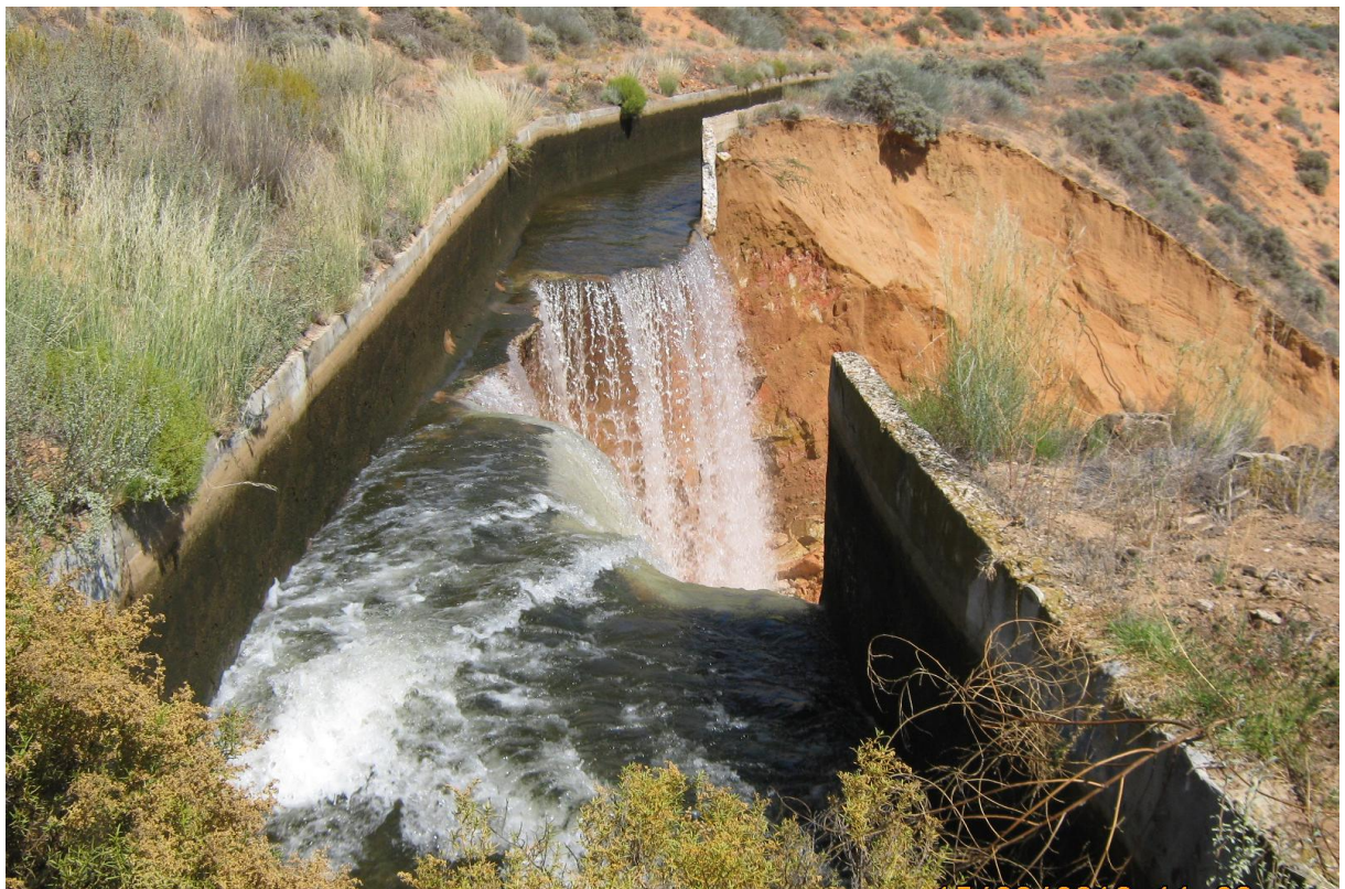
Figure 7-2: Major canal failure
