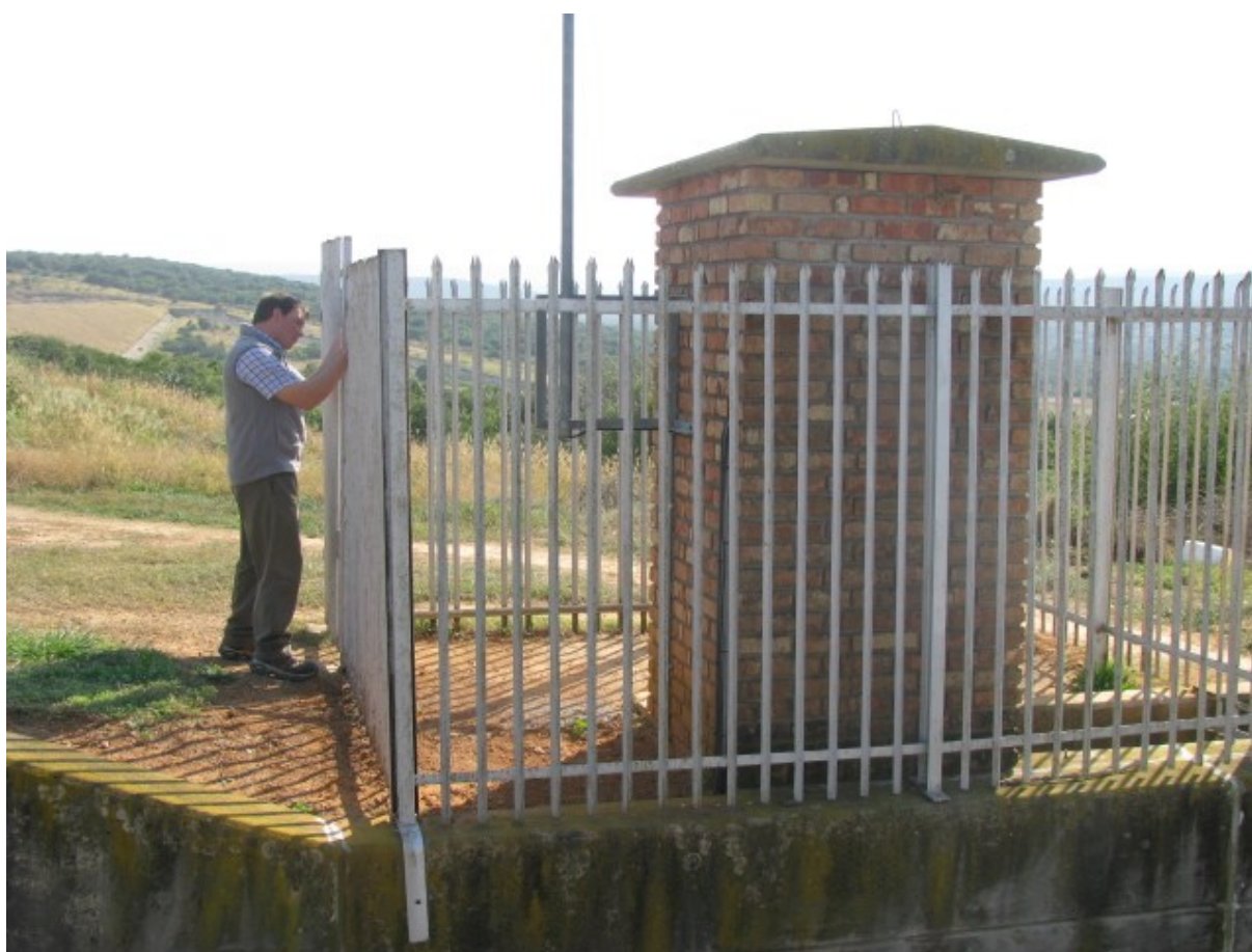
Photo 4:3: Telemetry system at the main canal downstream of Scheepersvlagte Dam
