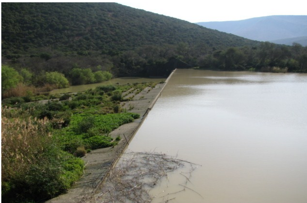
Photo 5:2: Photo of the fair condition of Korhaans weir
