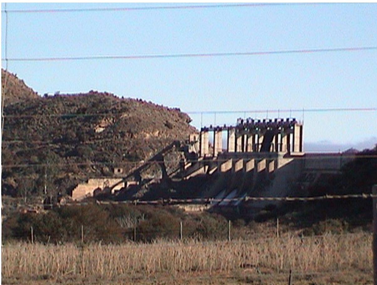
Photo 5:1: Dam wall of Darlington Dam
