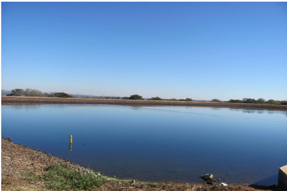
Figure 7-5 Balancing dam on the right bank
