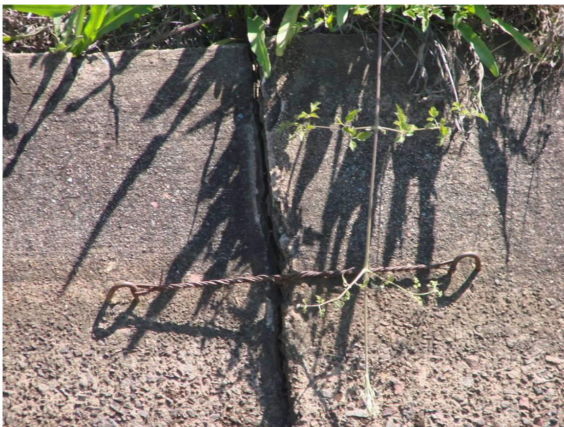
Figure 7-3: Temporary measures to stabilise canal
