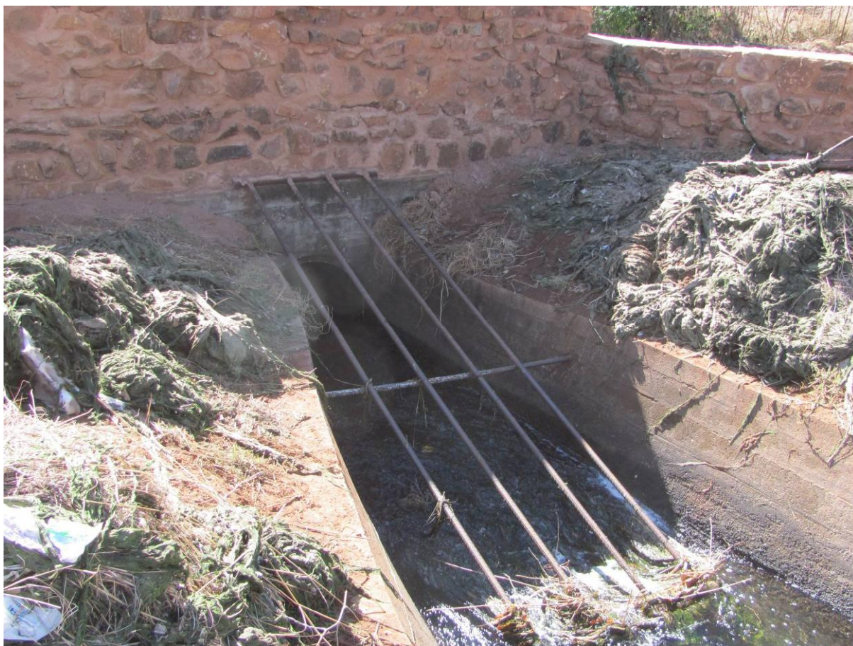
Figure 4-5 Entrance of siphon with screen
