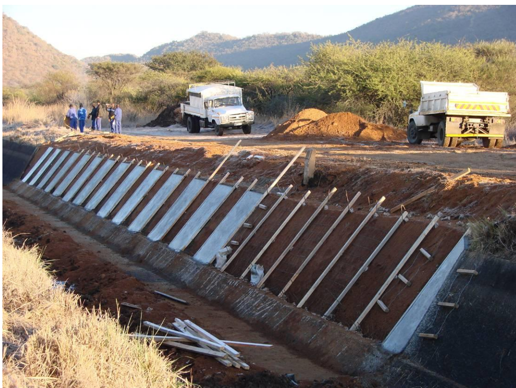
Figure 4-2 Restoration of canal sections on the left bank
