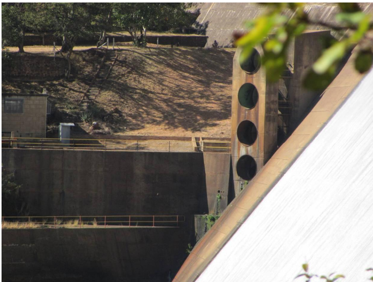
Photo 3-1: View of the Hereford outlet works at the Loskop Dam wall
