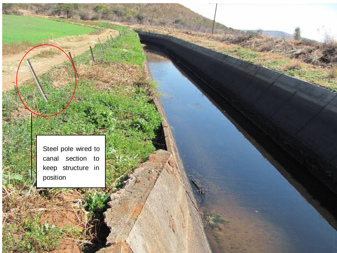
Figure 4-3 Canal stabilisation on the left bank
