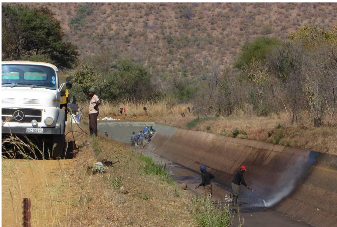
Figure 7-2: “Smooth and Patch” of canal section
