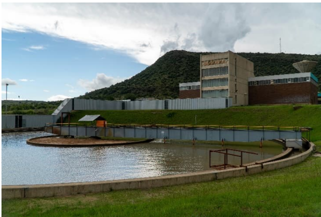
Figure 3-41: Primary sedimentation - clariflocculator
