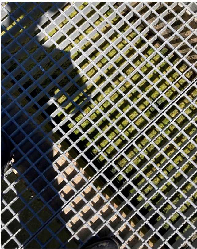
Figure 3-59: Algae scum in filter inlet channel
