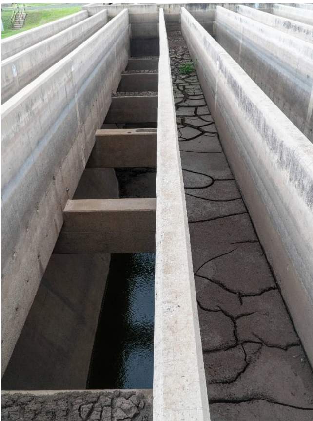
Figure 3-43: Primary sedimentation – horizontal flow system
