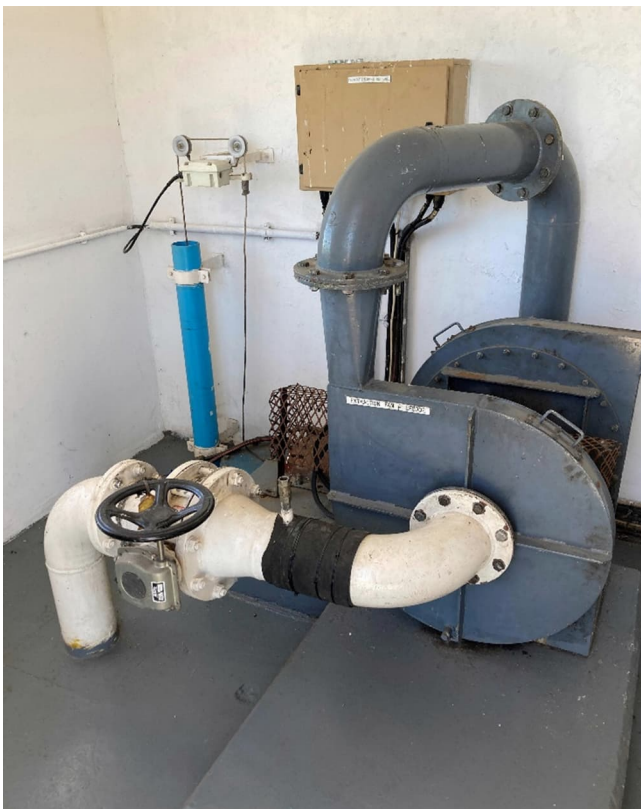
Figure 3-55: Pulsator vacuum pump (not operable)
