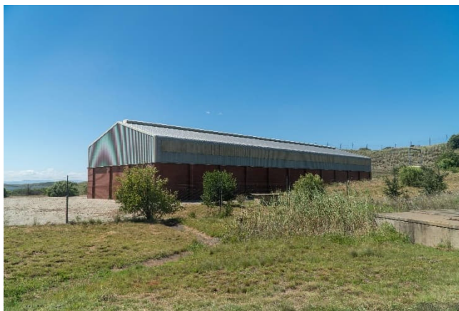
Figure 3-1: Novo Pump Station building
