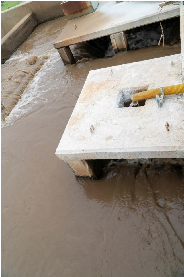
Figure 3-37: Lime dosing
