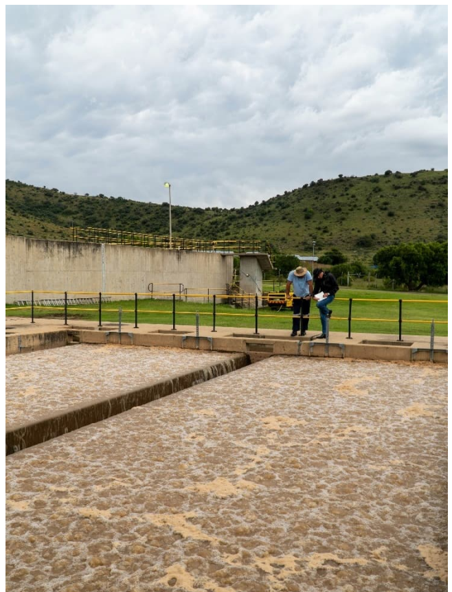
Figure 3-44: Filters backwashing
