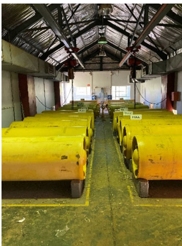
Figure 3-65: Chlorine drums
