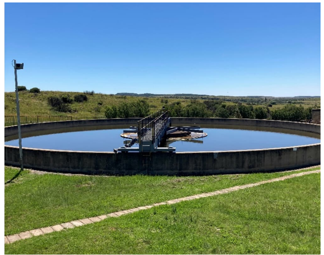
Figure 3-52: Turbo-circulator clarifier
