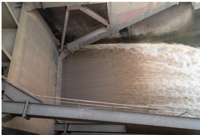
Figure 3-31: Sluice Gate 5 open
