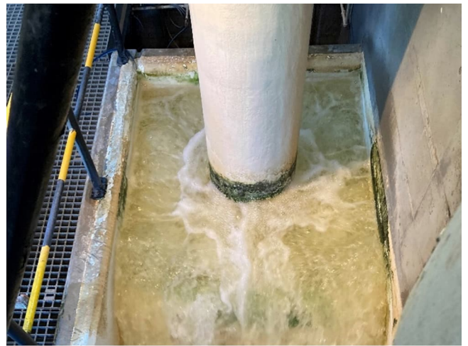
Figure 3-62: Filtered water inspection chamber (partialisation-siphon system over-aerating)
