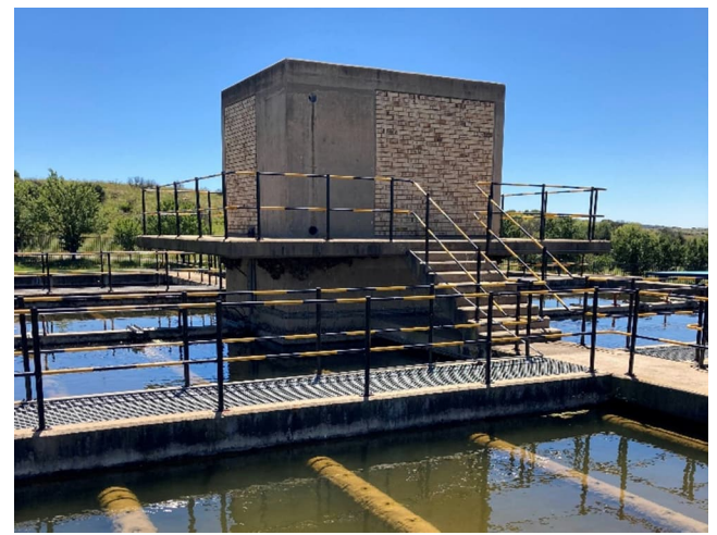
Figure 3-54: Pulsator vacuum control building
