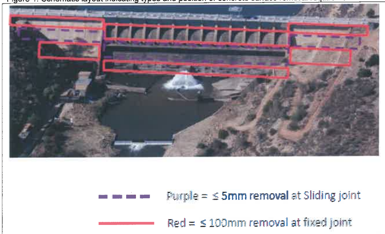
Figure 1: Schematic layout indicating types and position of concrete surface removal requirements
