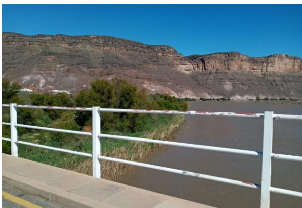
Figure 24: Site photograph (2024) obtained from the DWS Upington Regional Office
