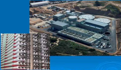
Palmachim SWRO plant is modular and easily expanded from 30 to 60 Mm 3 /Year
