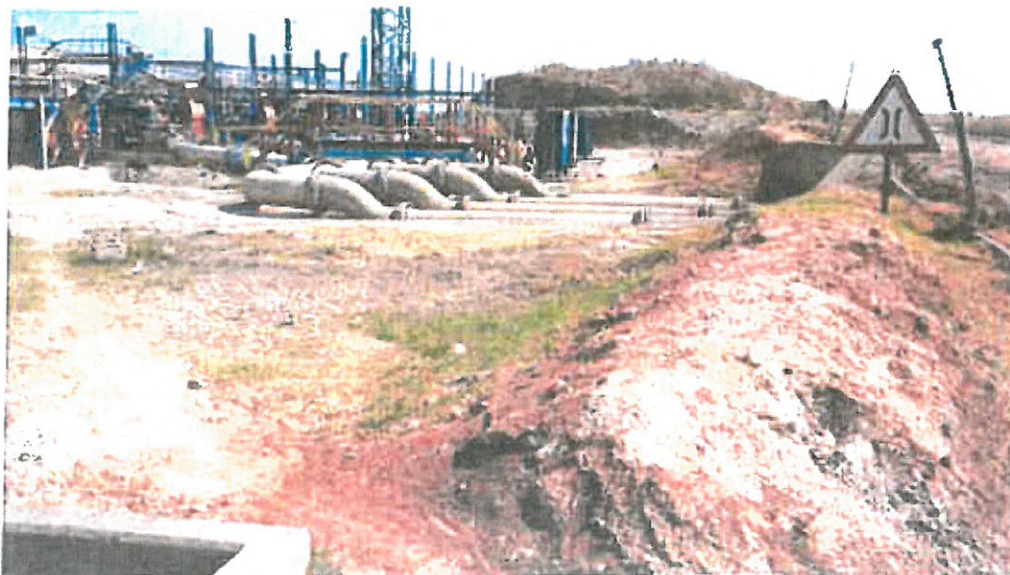
Figure 14: Rolled edge constructed to protect pump station and office
