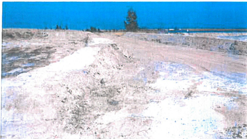
Figure 18: Temporary storm water containment next to return water dams (till East Storm Water Dam constructed)
