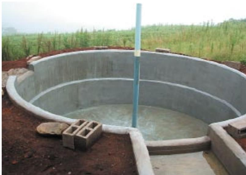
Figure 3: Typical 30 m<sup>3</sup> rainwater tank
