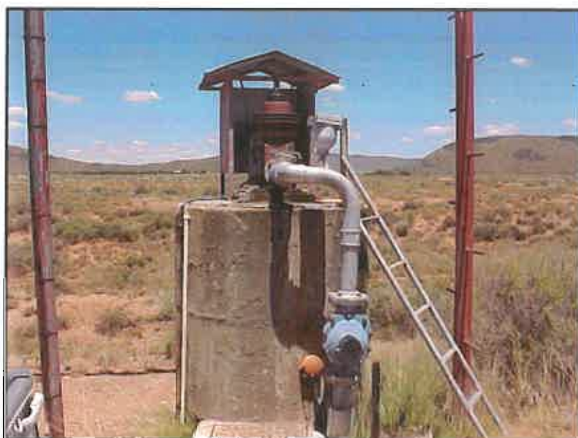
Plate 3: Production Borehole G23205F ('Suidwes' No. 7) in the South-Western Scheme, with cement platform to avoid damage to the hole and pump equipment during flooding (photo F. Fourie)
