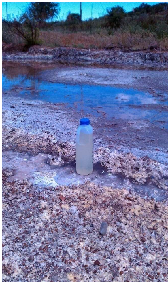
Photo 4-3: Salt precipitating north of the tailings dam where seepage decants
