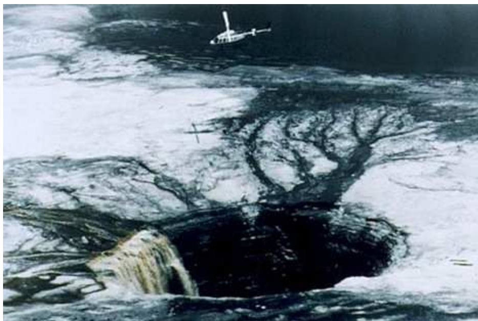
Photo 5-2: This sinkhole formed in 1994 inside a similar gypsum tailings dam in Florida
