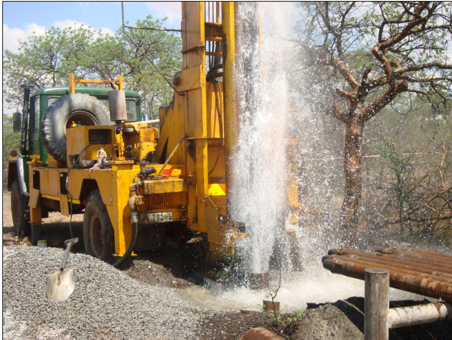
Photo 3. Borehole with blow yield in excess of 40 l/s drilled on the Farm Brilliant south of Senwabarwana (Photo taken by Martin Holland).
