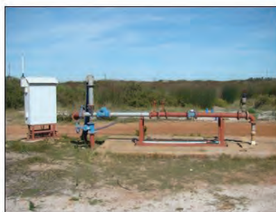
Abstraction wellhead in the Atlantis wellfield
