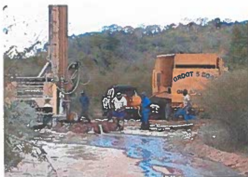
Figure 3 : The rotary air percussion drill rig
