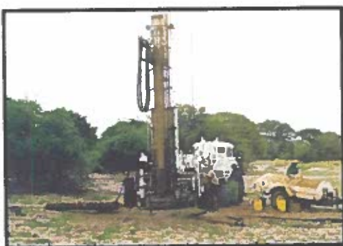
Figure 3 : The rotary air percussion drill rig.
