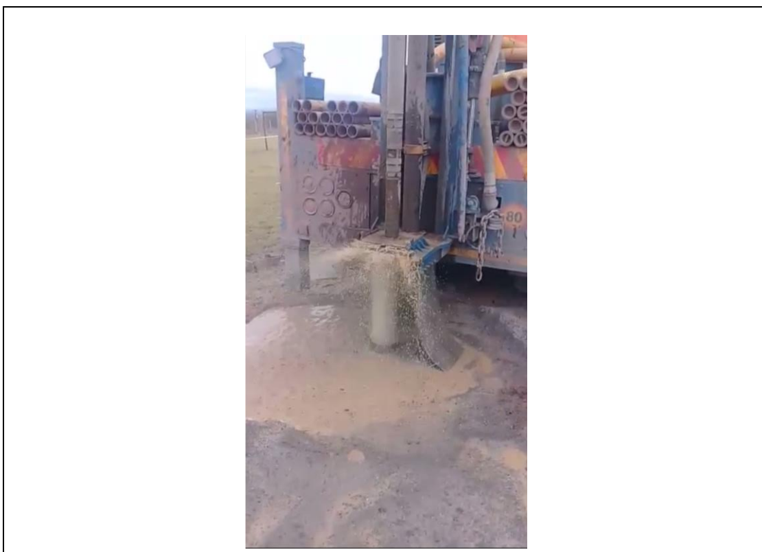
Figure 4-1: Drilling at Isinyabusi Technical High School
