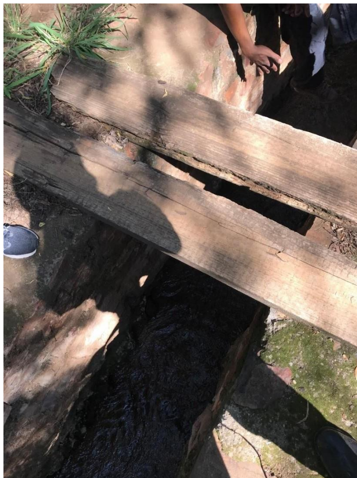
Figure 26 The concrete furrow where water from the Broederstroom spring collects as it flows downstream
