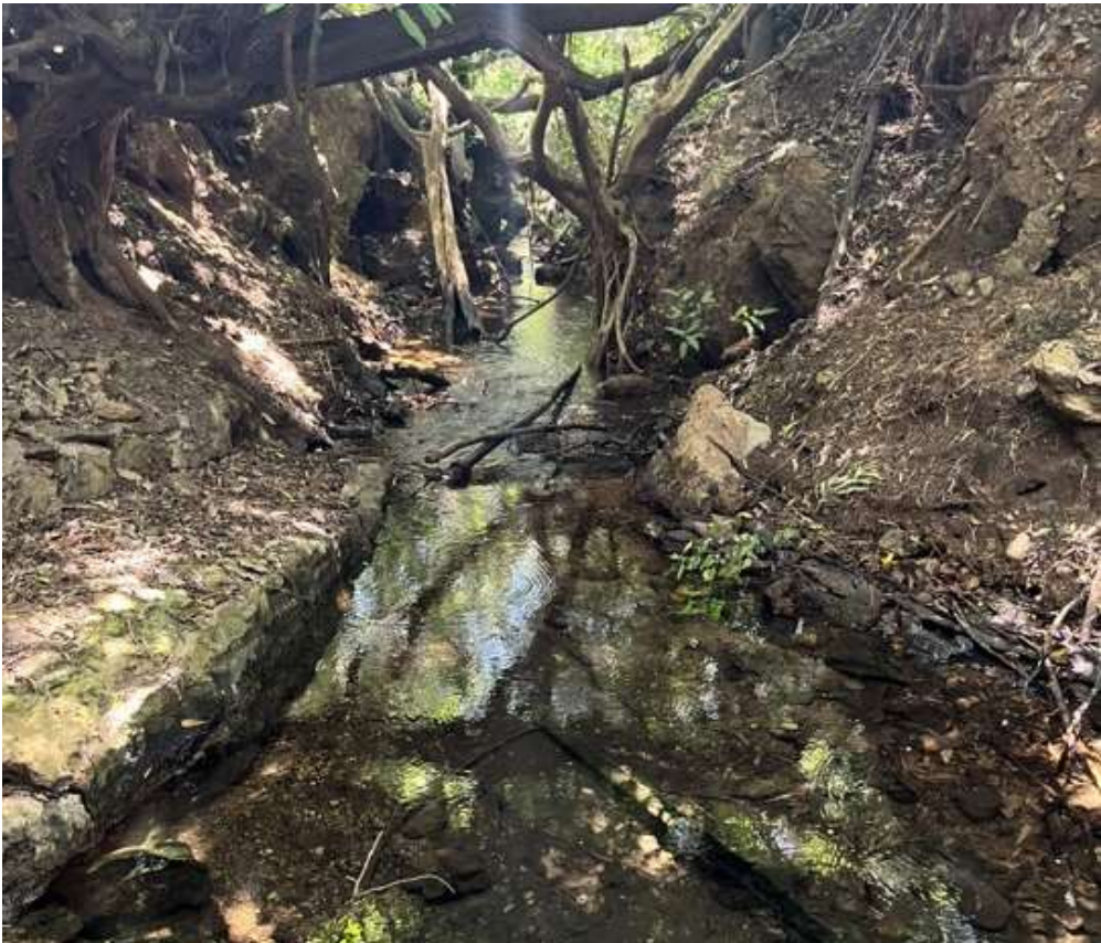
Figure 24 The concrete furrow near the eye of the Broederstroom spring where water collects as it flows downstream
