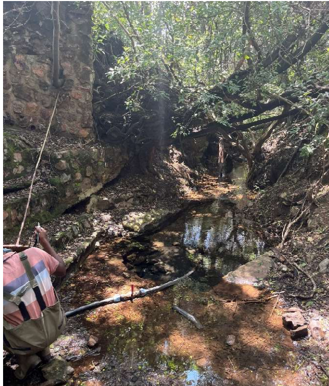
Figure 26 The concrete furrow near the eye of the Broederstroom spring where water collects as it flows downstream
