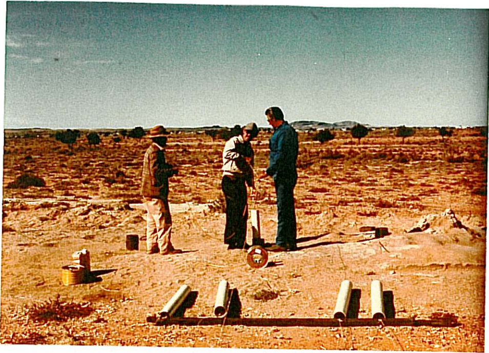
PLATE 8: Lowering the charge to the required depth in G34348, Site 3
