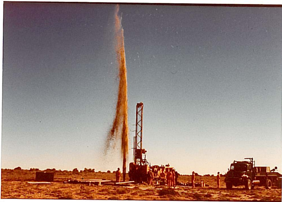
PLATE 12: Significant interconnection between two neighbouring boreholes at site 3 after blasting, as evidenced by this attempted 'blow test'
