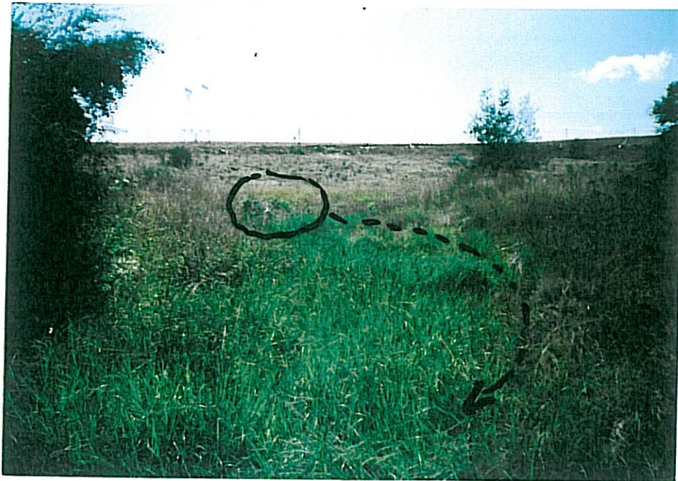
Discharge point at Spring No 2.
