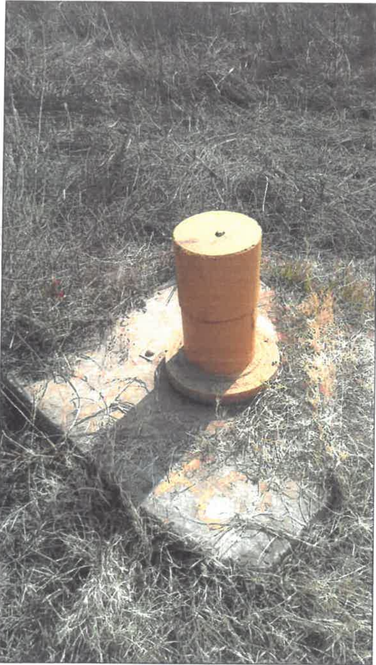
Photo 3: View of the A2N0640 borehole site.
