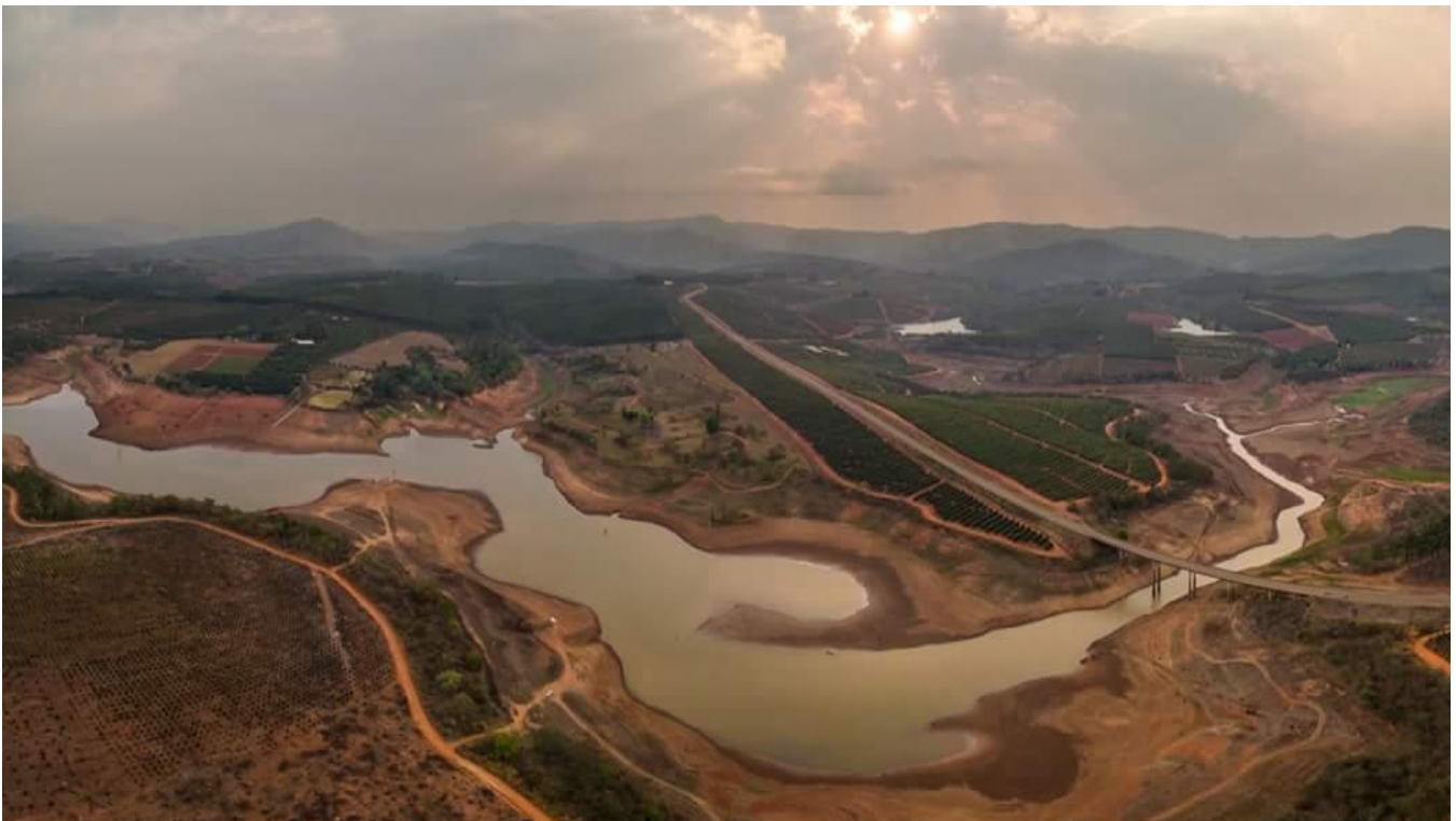
Tzaneen Dam: Photo courtesy of Willie and Mariette Botha
