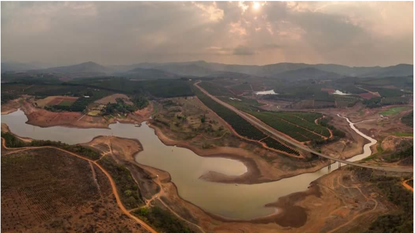
Tzaneen Dam: Photo courtesy of Willie and Mariette Botha
