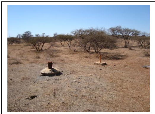
Photo 2-1: Borehole drilled 72m and 120m in the Hout River and Goudplaats Gneiss in the Limpopo Province respectively
