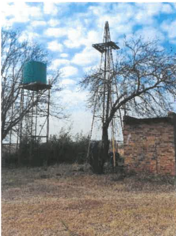
Photo 3: View of C2N0104 existing site.
