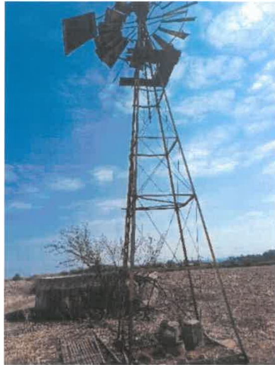
Photo 2: View of C2N0002 existing site.
