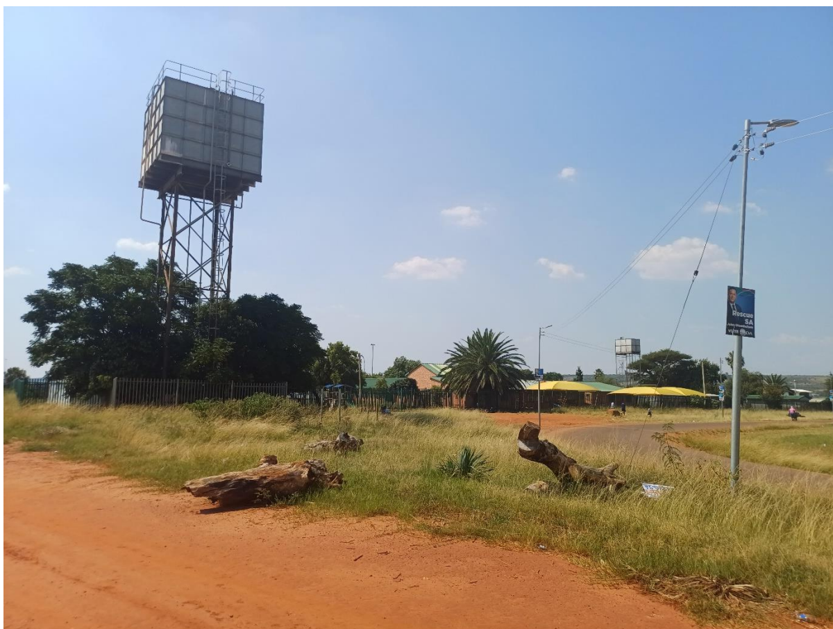
Photograph 1: View of the Slimline Steel Water Tank at Primary School
