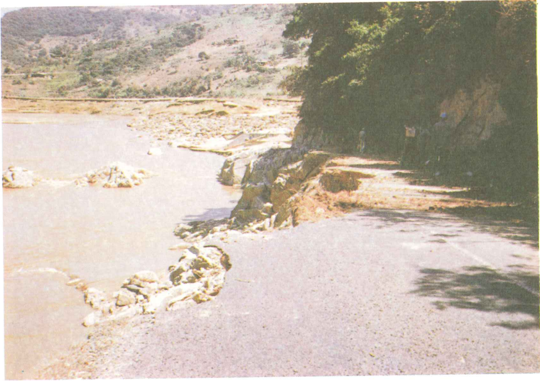
53. Mvoti River: lateral bank erosion on the outside of a bend, destroyed the road
