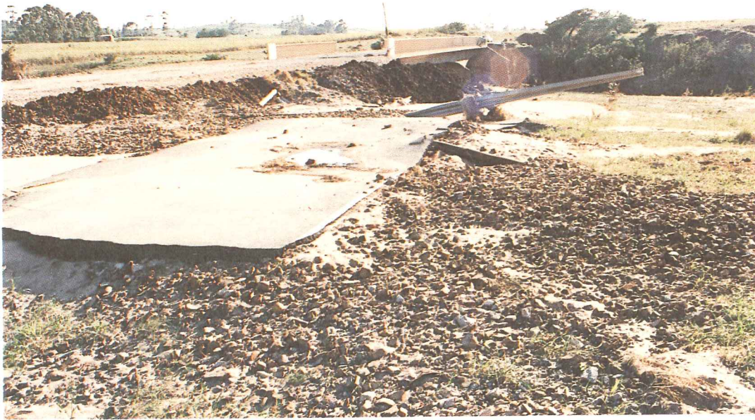
65. Nyezane River: bridge on N2 viewed from right bank. The asphalt surface in the foreground was carried intact off the road surface
