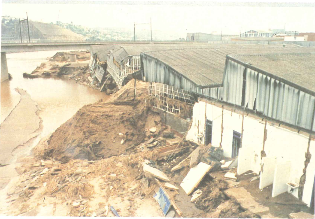
47. Damaged factory premises adjacent to the Mgeni River. Damage due to collapse of river banks. Deposition in factory was approximately 2m deep
