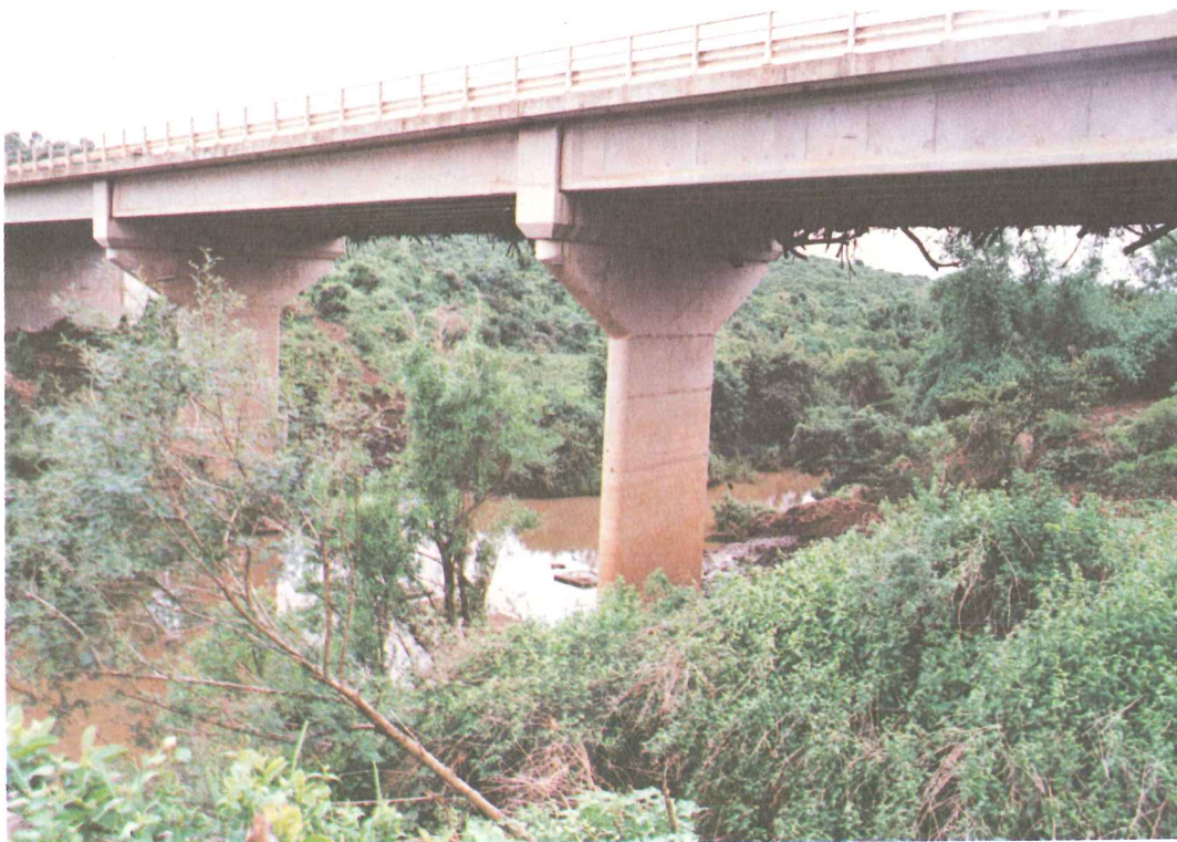
74. Nyalazi River: Site 93. Note debris trapped under the 13,2 m high bridge deck
