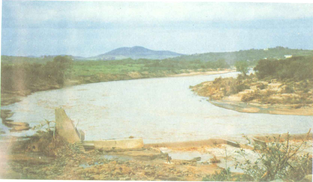
67. Mhlatuze River: Site 80, destroyed gauging station W1M09 and extensive scour of the right bank
