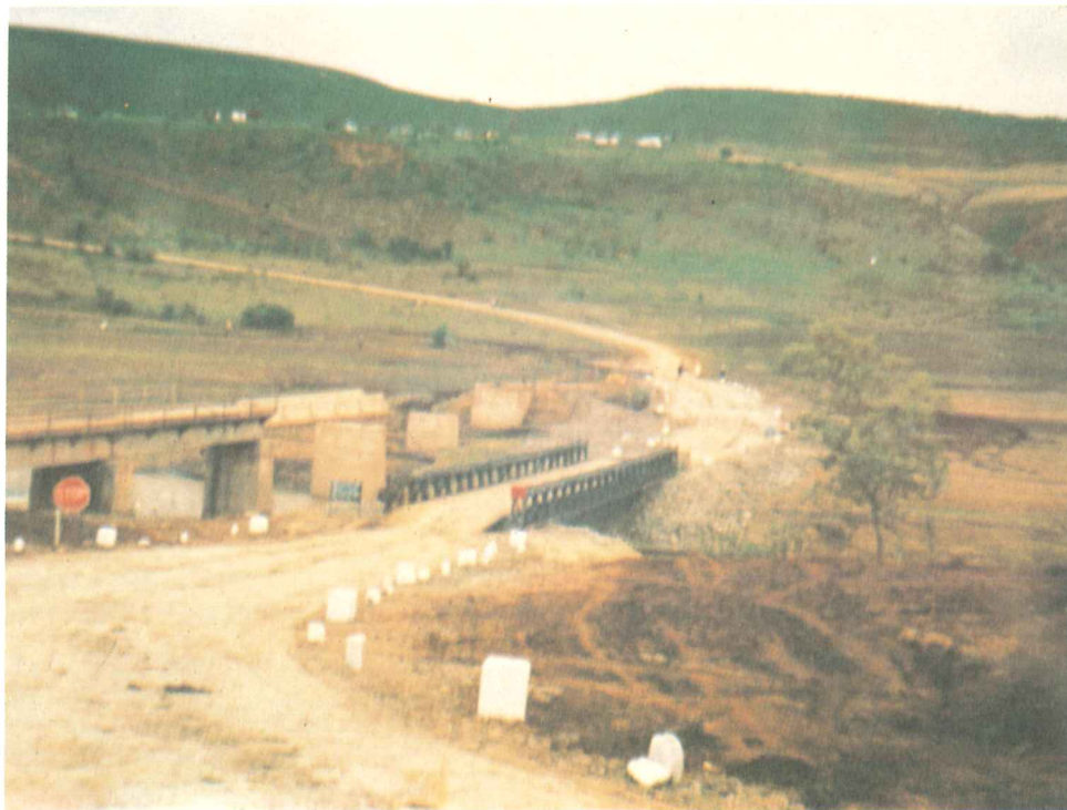
18. Mtamvuna River: upstream of Site 3, bridge at Gundrift, deck on south side washed away
