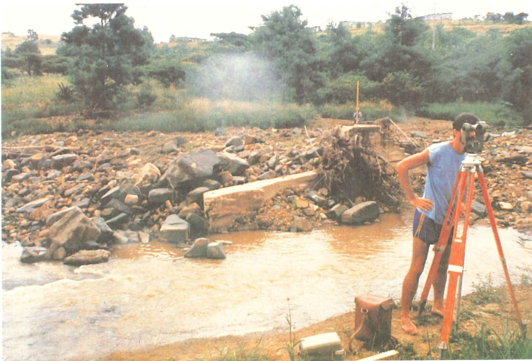
66. Mfulozane River: Site 78, gauging station W1M05 destroyed due to river course change
