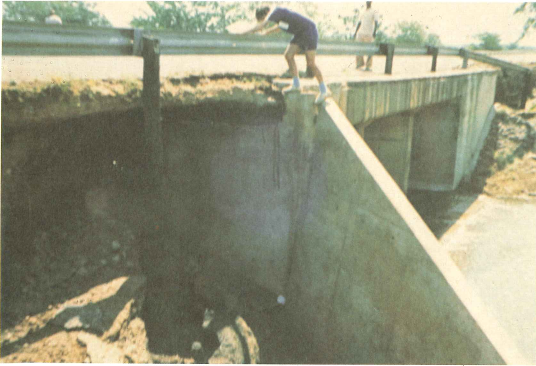
75. Mzinene River: Scour of approaches along the downstream side of the N2 bridge, between Hluhluwe and Mkuze. The flow was 0,3 m deep over the bridge deck
