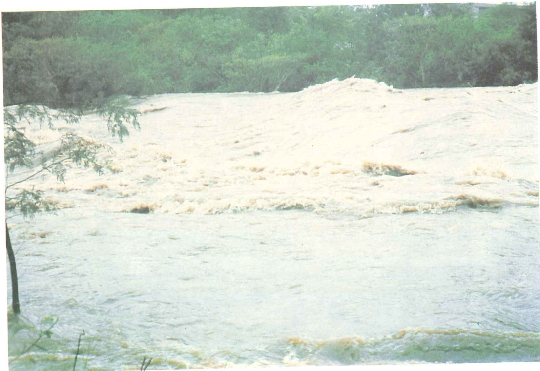
30. Mgeni River: at U2M01 upstream of Howick Falls, during peak. The weir is located below the wave in the foreground indicating critical to super-critical flow
