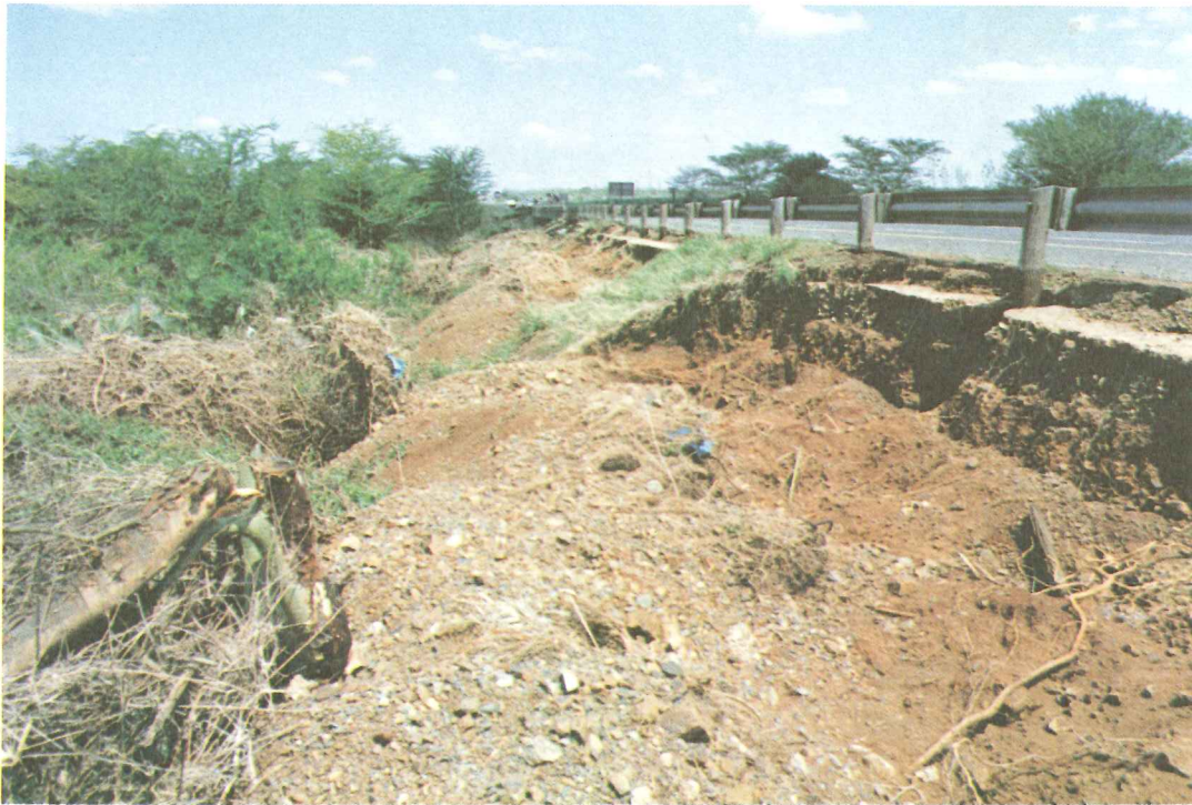
76. Typical scour behind the wingwalls on the downstream side of the N2 bridge crossing the Ncemanne River
