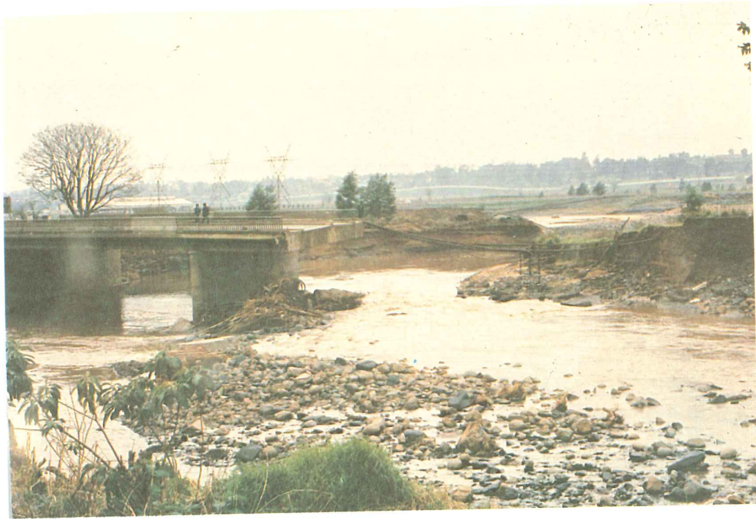
37. Msunduze River: Edendale bridge in Pietermaritzburg, failed due to river course change
