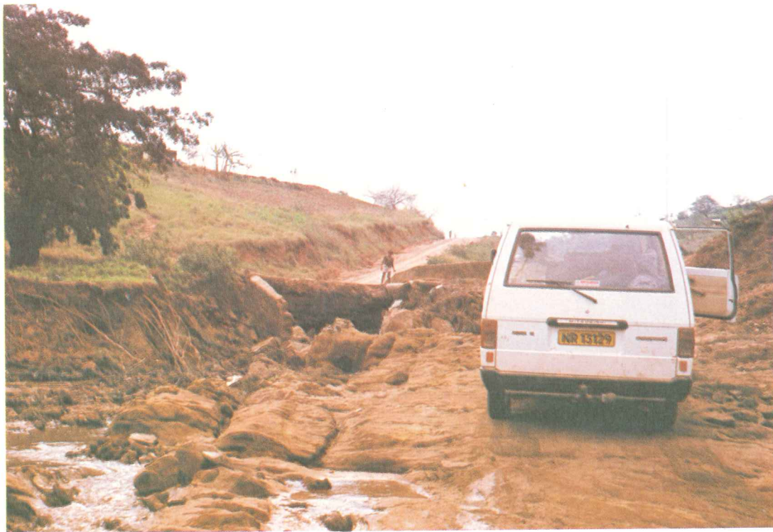
34. Typical gully erosion on rural road in the Mgeni River catchment at Nagle Dam
