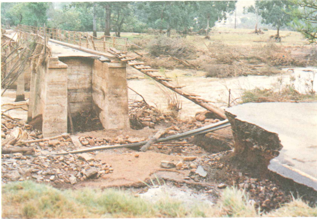
33. Single carriage bridge downstream of Albert Falls Dam, on the Mgeni River. Although both approaches were breached, the main structure did not suffer any significant damage
