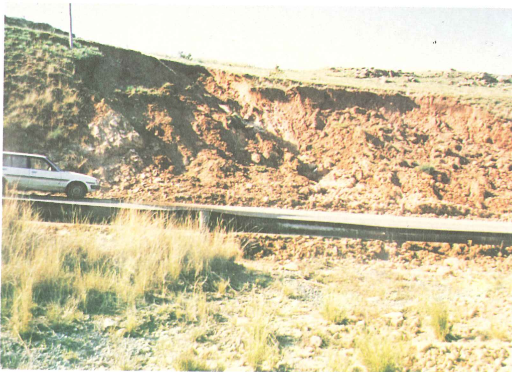
56. Slip in road cut along the road between Kranskop and Mapumulo
