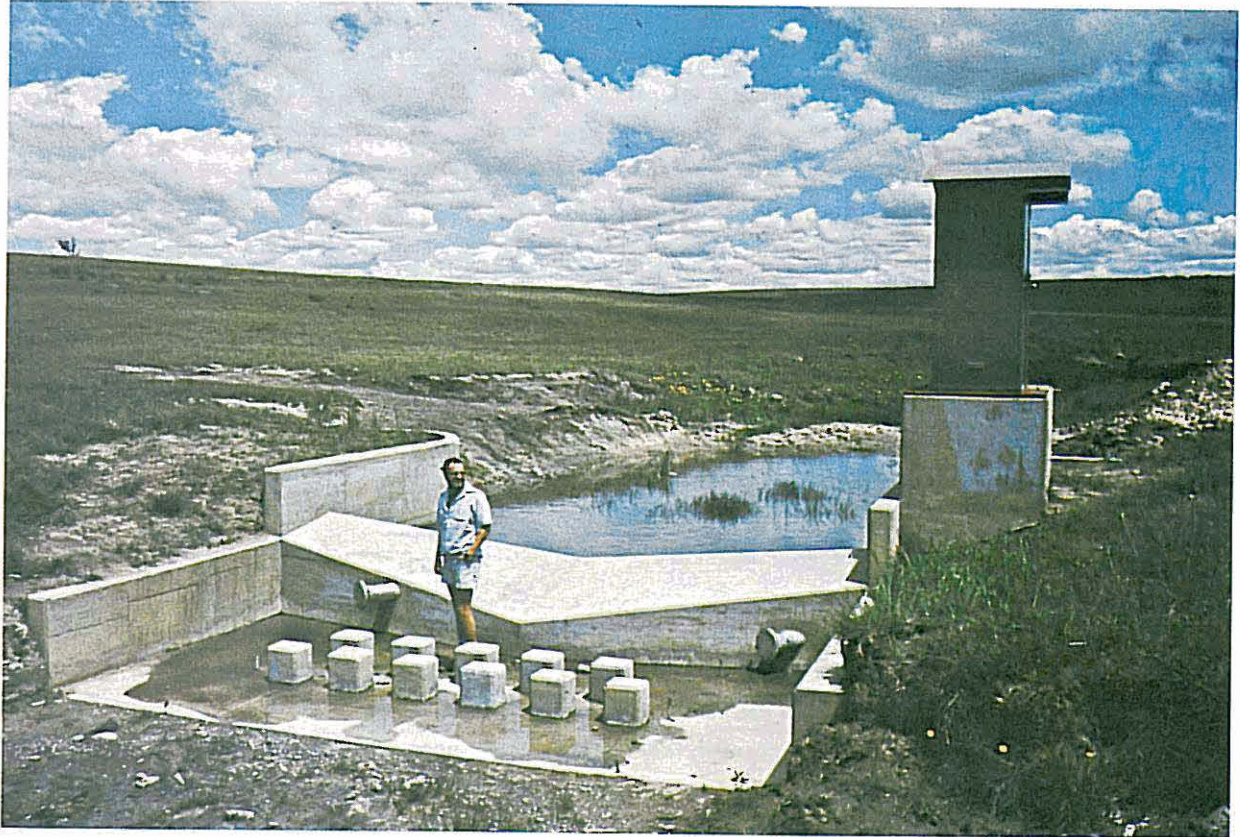
PLATE 1: Crump weir at C8M25
